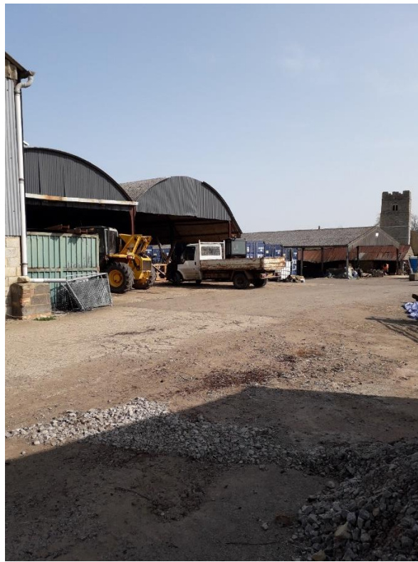
View within farm complex showing church tower
