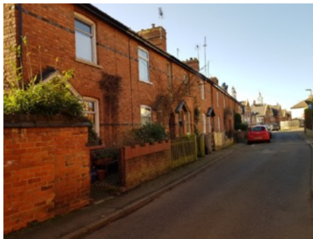
Fig. 18: The former Board School from Bury Street, the three roof lanterns are a notable feature in the surrounding street views. (SGA 2020)
