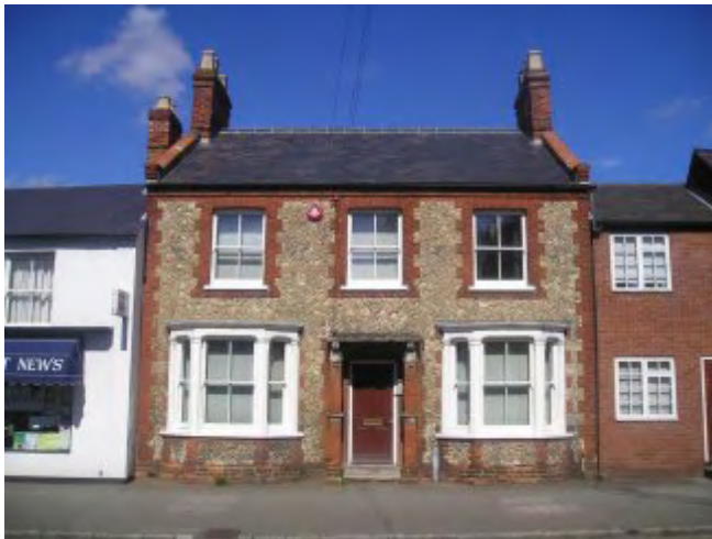
Picture 28 A handsomely proportioned house with Welsh slate roof, brick dressings around the upper windows and timber canted lower bays either side of the central door. The stone coursing is intended to convey a robust rustic character to the house
