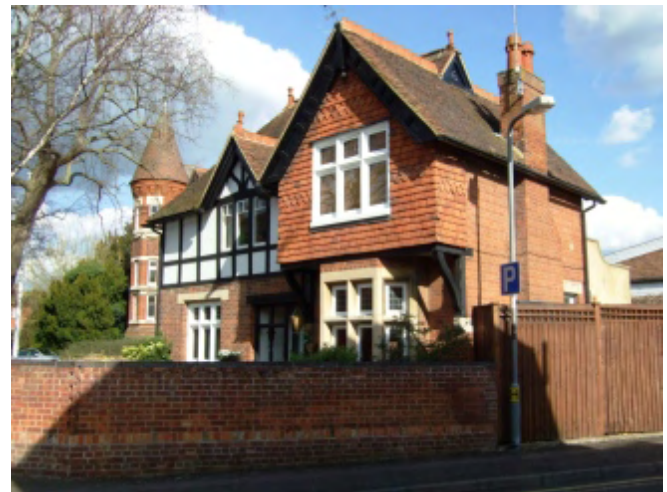
Picture 24 The Lodge, Lovat Bank: Clay tile roof, fancy ridge tiles with finials; ornamental, tile hung, cantilevered, first floor front wall; stone canted bay; stone cills and lintels; timber bargeboards and applied 'timber frame' and roughcast decorative detail
