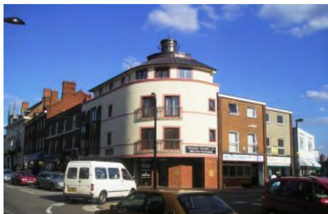
Picture 32 Contemporary development in the conservation area
