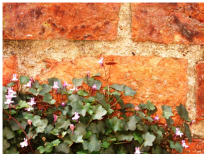
Picture 27 Lime pointing (minerals in the lime will encourage plants to grow; creepers such as ivy should be discouraged, however)
