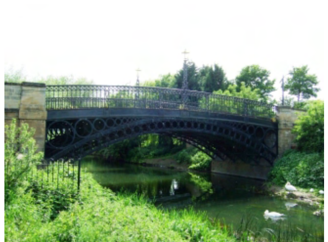
Picture 15 Tickford Bridge
