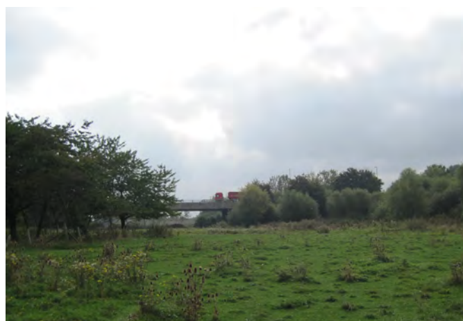
View of elevated A509 looking south from within site
