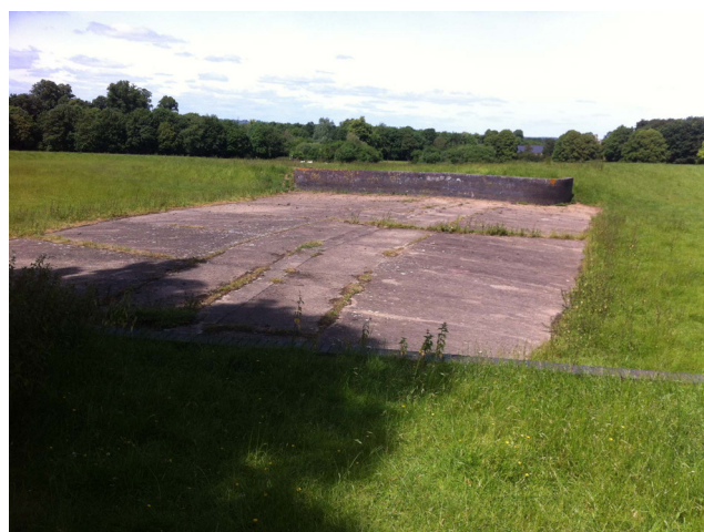
Existing infrastructure associated with the balancing lakes nearby.
