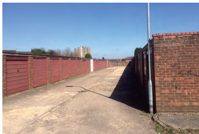
The site comprises of residents garage parking area.
