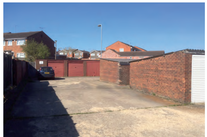
Road serving three rows of garages
