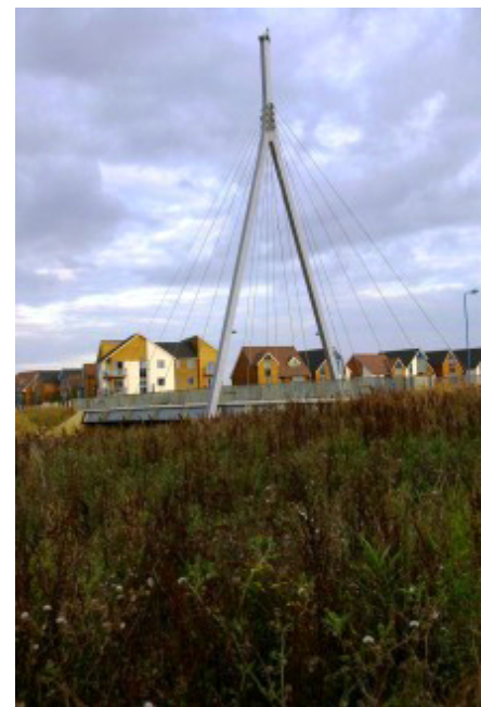
Picture 9 The new bridge over Broughton Brook is a prominent and memorable local landmark
