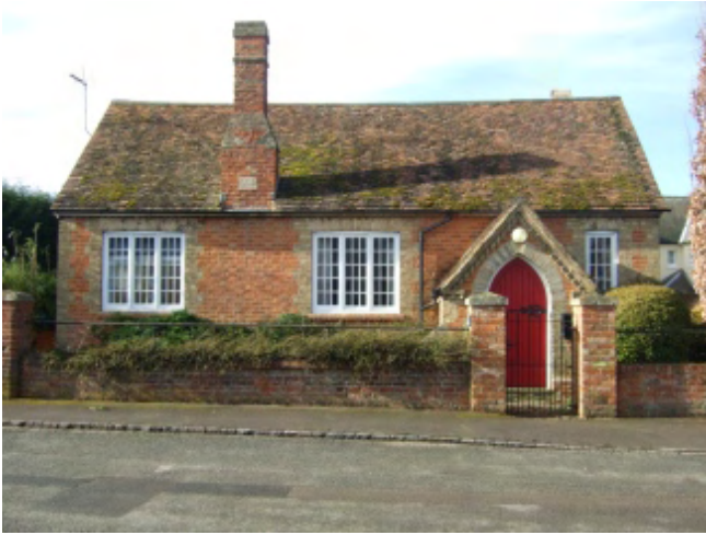
Picture 7 Clay tile, brick, stone, timber and iron used in a harmonious combination at the Old School House
