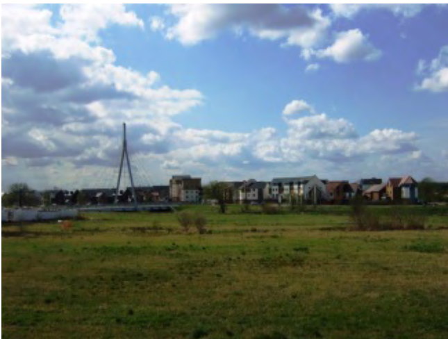
Picture 2 View of new bridge over Broughton Brook with housing under construction beyond
