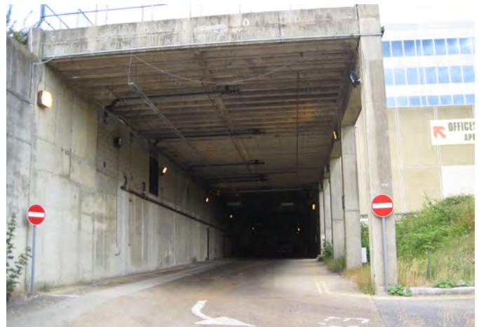
Service road serving CBX
