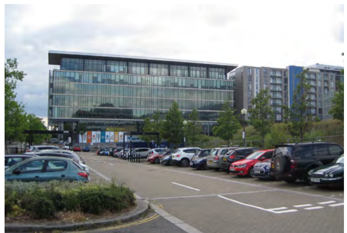
View looking west towards The Hub
