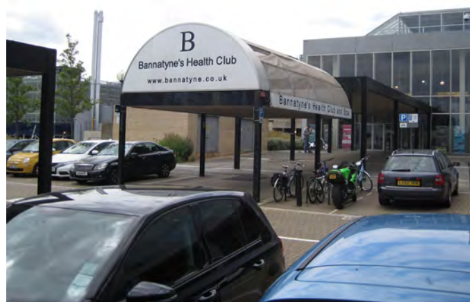
Entrance to CBX adjacent to the site
