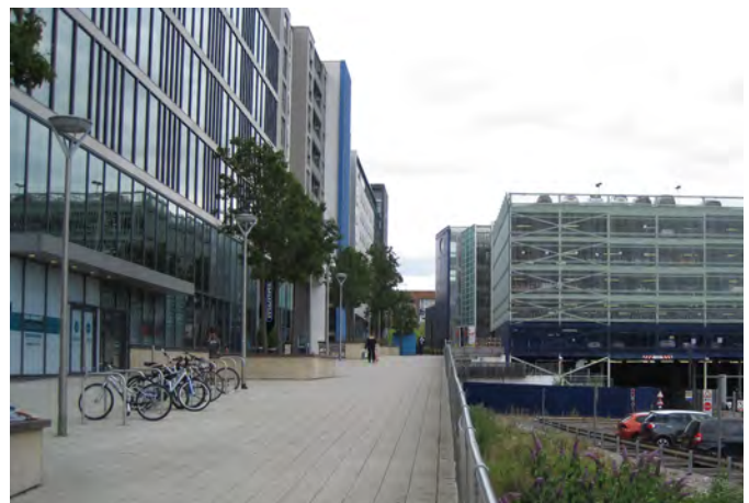
Raised pedestrian route adjacent to eastern edge of The Hub
