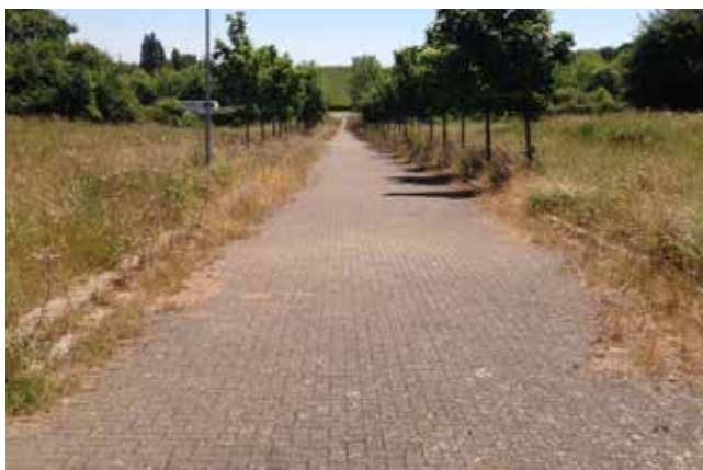
Existing infrastructure within the site
