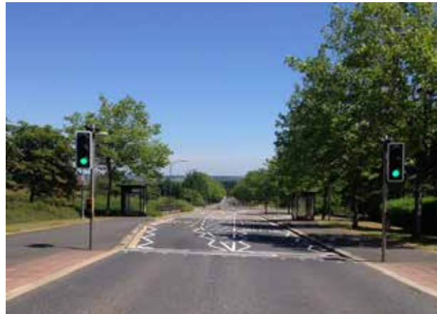
Example of alternative treatment on Silbury Boulevard to facilitate pedestrian crossing
