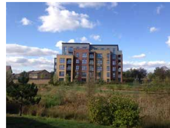
Example of a contemporary building in a landscape setting
