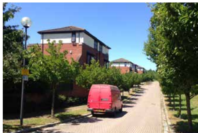
Existing housing on Adelphi Street and avenue of trees along western edge of site. These trees should be retained.
