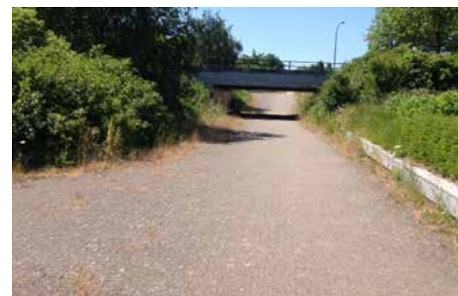
Redway and existing underpass underneath Skeldon Gate which runs alongside the southern edge of the development sites
