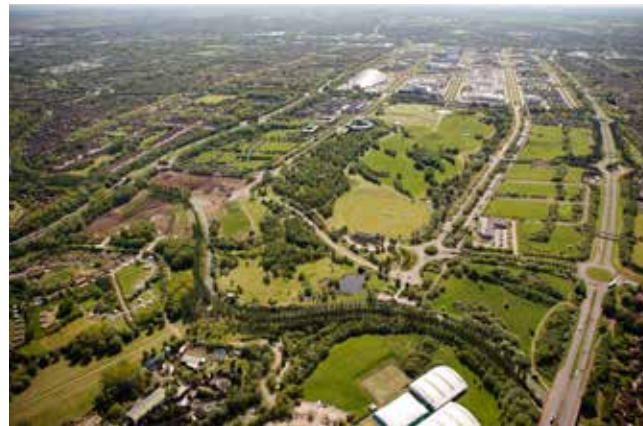
Campbell Park Northside with adjacency to the city centre, Campbell Park, the Grand Union Canal and Newlands
