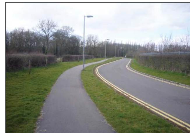
fig 17 Vehicular access to Newlands site off Frobisher Gate
