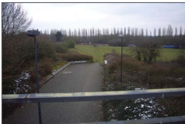
fig 16 Existing pedestrian underpass into Campbell Park site from Avebury Boulevard
