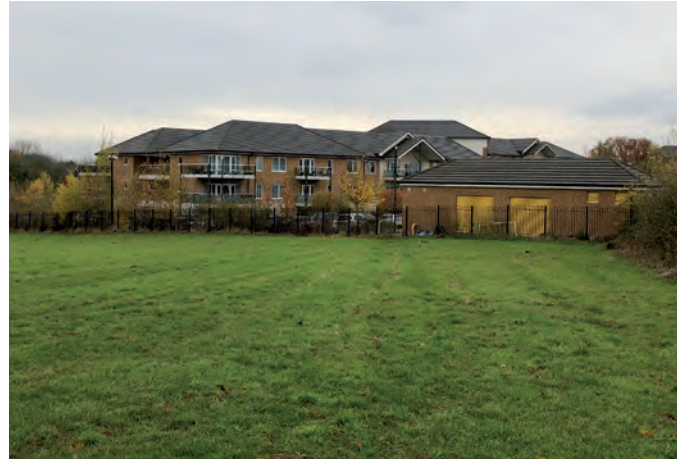
Surrounding building types illustrating buff brick and pitched roofs with balconies, some painted timber cladding and glazed atriums.
