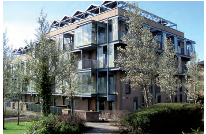
Example of a key building with balconies creating an active frontage
