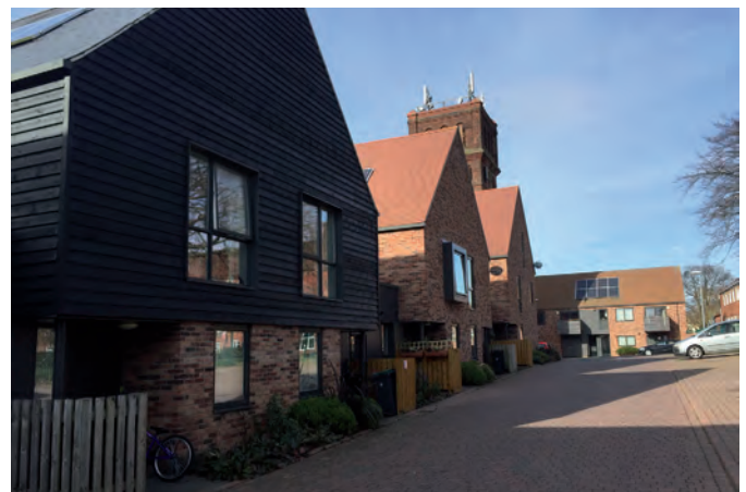
Gable ends addressing the street can create a strong built form presence
