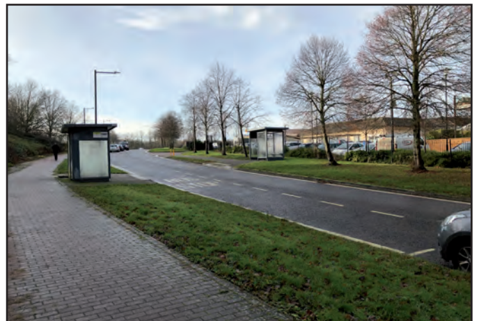
Bus shelters on Chalkdell Drive
