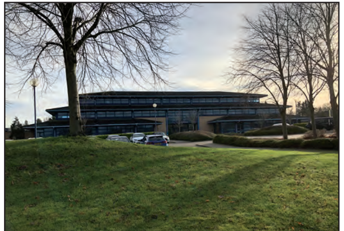
View of pavilion buildings from redway on Chalkdell Drive
