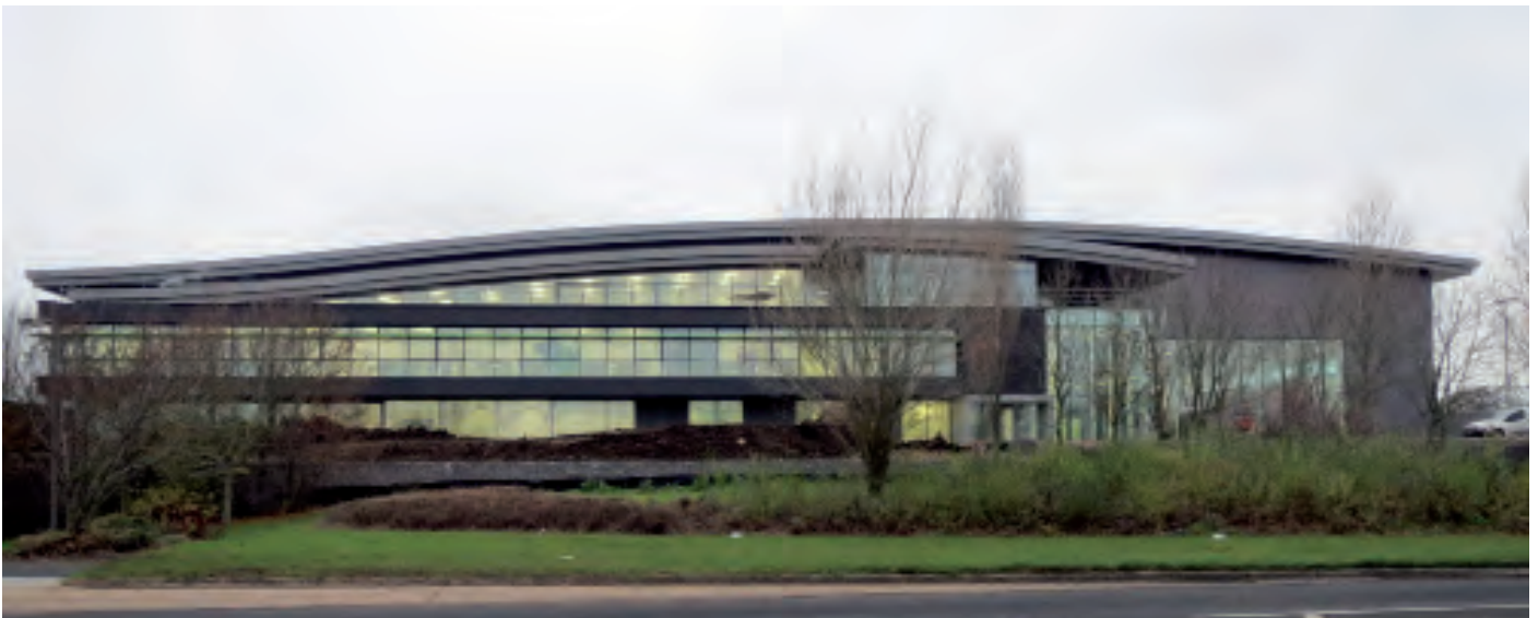
Well considered windows in employment buildings can add character whilst increasing surveillance of private and public spaces
