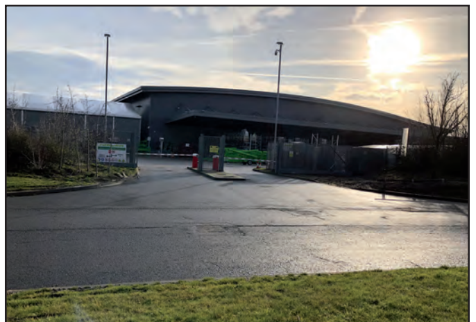
Nifty Lift HGV Service access on Foxcovert Road.
