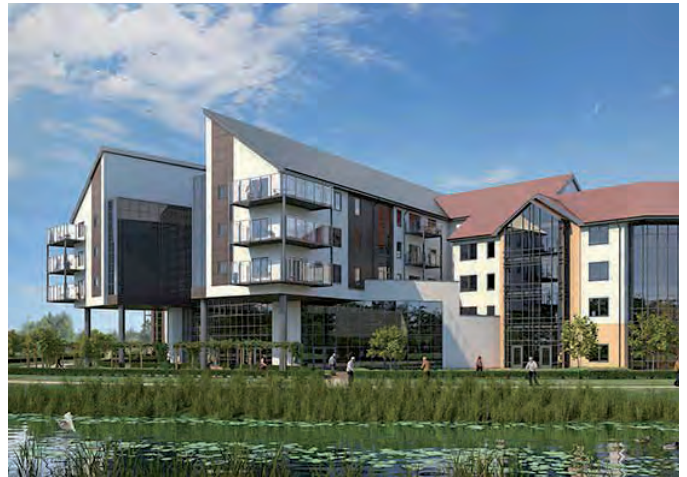
Example of well considered C2 residential development taking full advantage of landscape features
