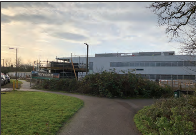
View of newly constructed powertrain HQ on neighbouring site from Redway on Foxcovert Road
