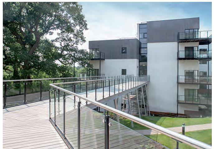
Open air access to surrounding landscape within development parcel provides interest and character
