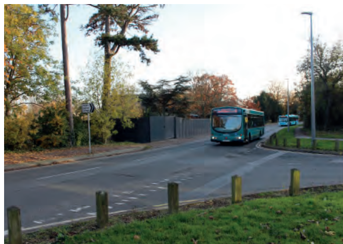
View south along Sherwood Drive with former Fire Station behind temporary fencing
