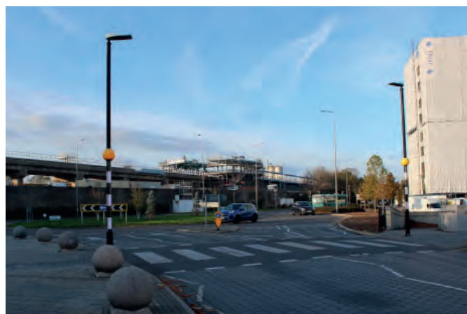
View of Brunel Roundabout with transfer building for East West Rail under construction
