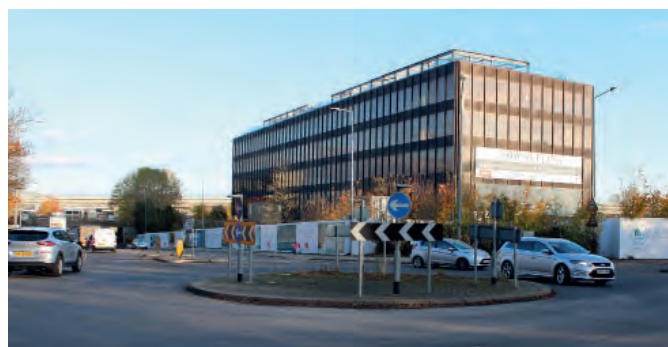
Former office building to south of site being converted into apartments (Caspian View)
