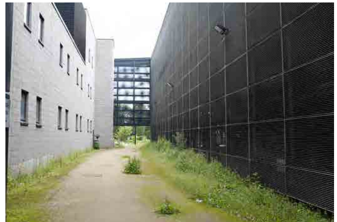
View of service access path to rear of the theatre along northern edge- It is publicly accessible but highly unattractive.
