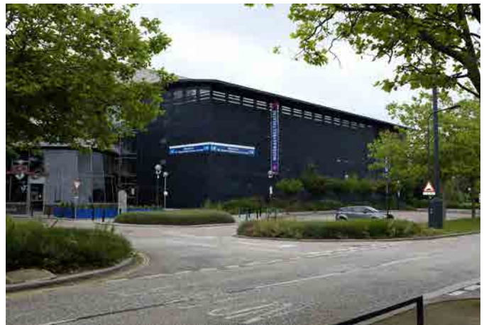
Classic CMK Infrastructure to the east of the Theatre Car Park .
