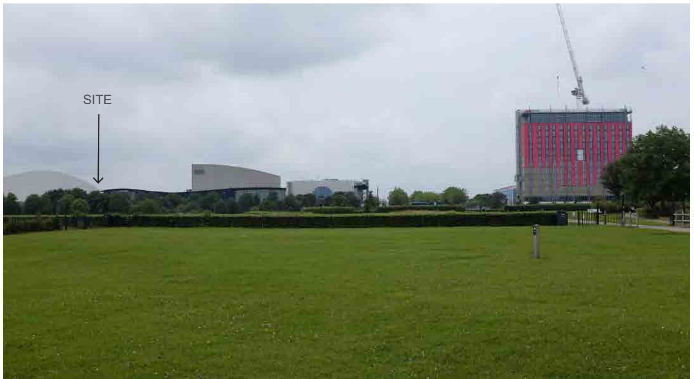
View of site in current skyline from Campbell Park
