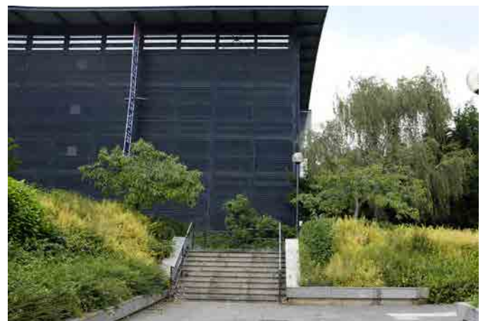
View of east corner of the site from the underpass under Avebury Boulevard
