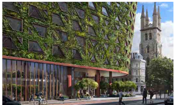
Example of how biodiversity can be integrated to the fabric of a building and enhance its visual appearance.
