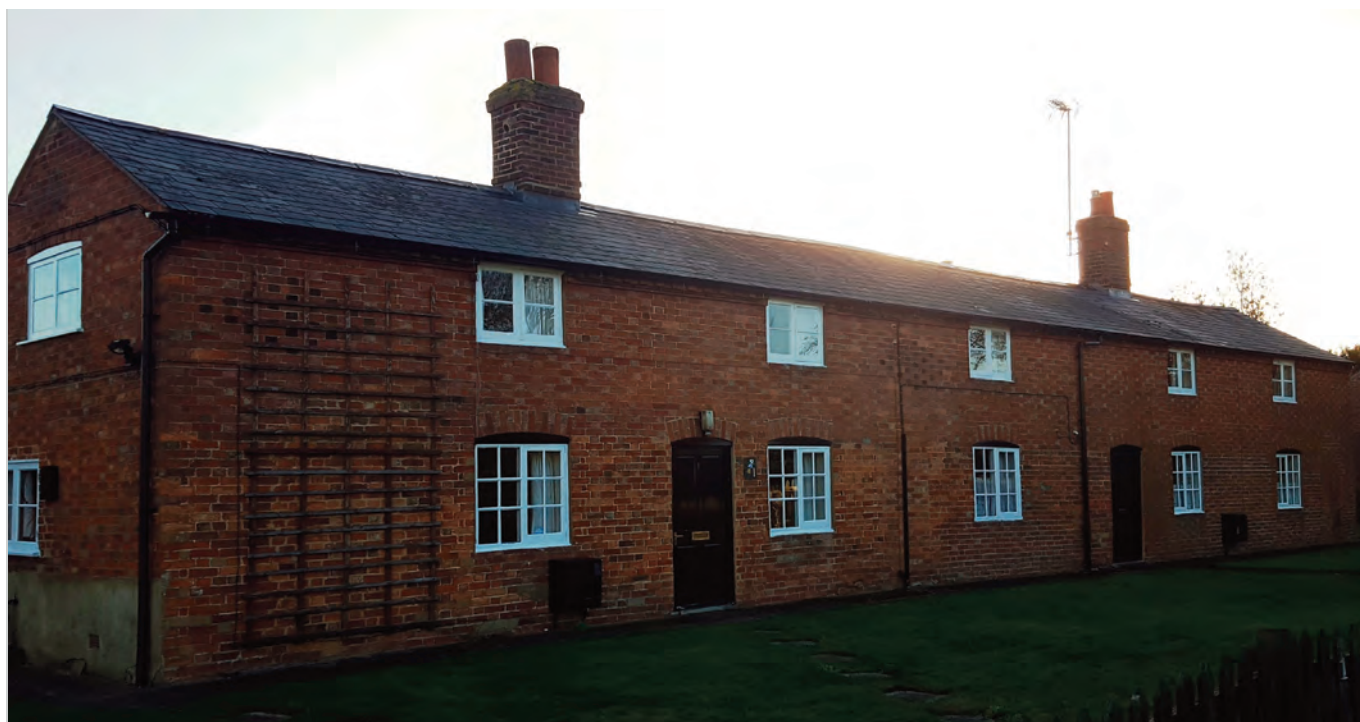
Brick terraced cottages with Welsh slate roofs and timber casement windows overlooking Broughton Rd
