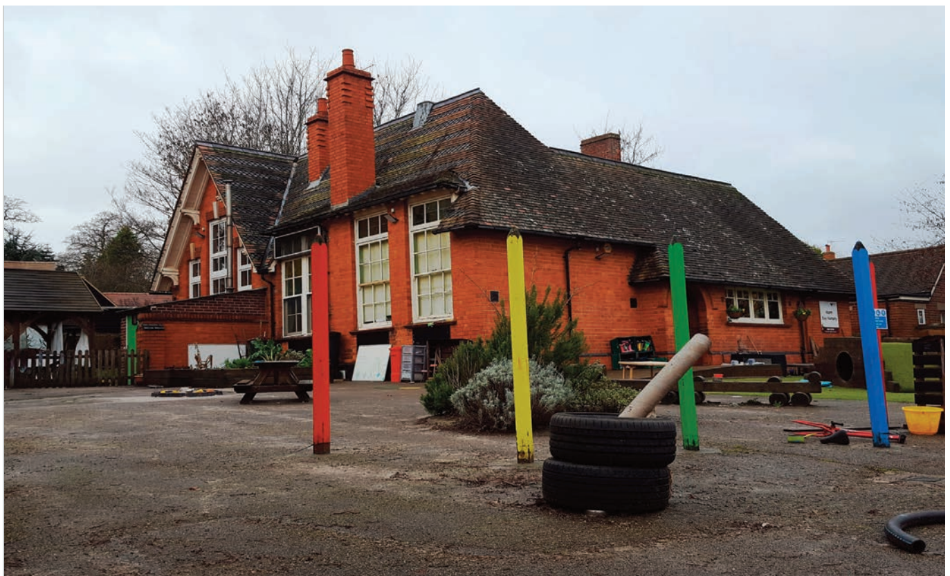
Former School Building, Shenley Church End
