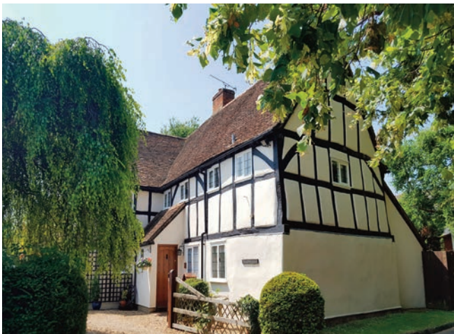
Timber frame Dower House, Shenley Road, Shenley Church End
