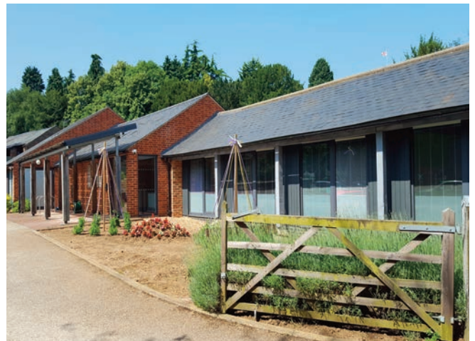
Refurbished barns adjacent Manor Farm House, Shenley Road, Shenley Church End
