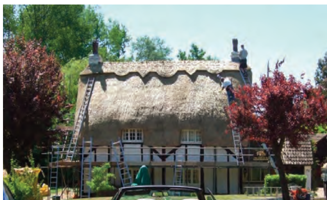
Rethatching at Freefolk Cottage, Church Green Road. The pronounced decorative ridge is not a traditional detail of the area.
