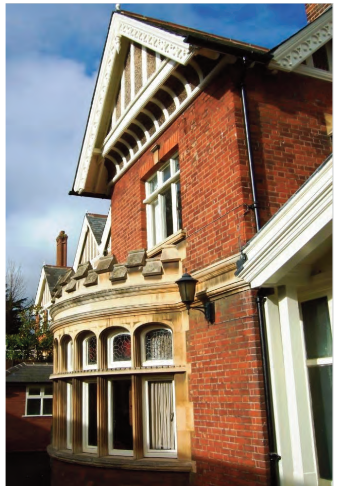
Stone, brick, timber, roughcast, lime mortar, lead and iron used harmoniously on a wing of Bletchley Park House
