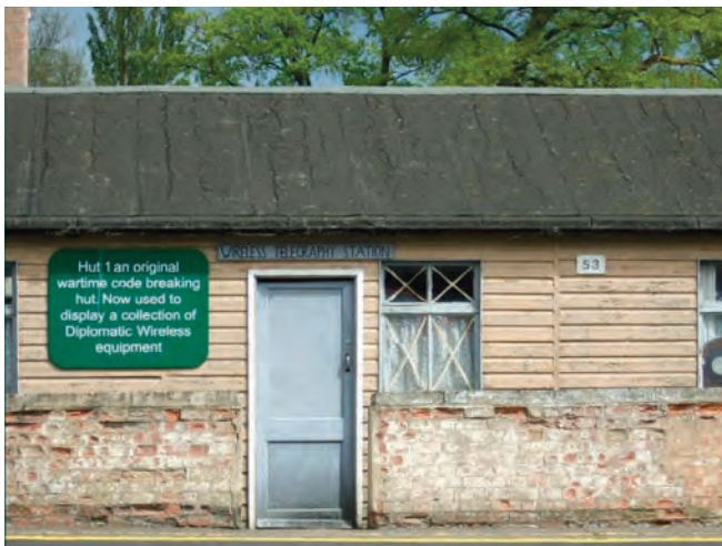
Hut 1, ship lap timber with remnant of blast wall in front and bitumen coated timber roof.
