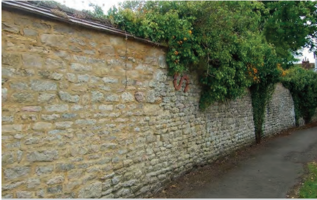
A tall boundary wall in stone with clay tile copings
