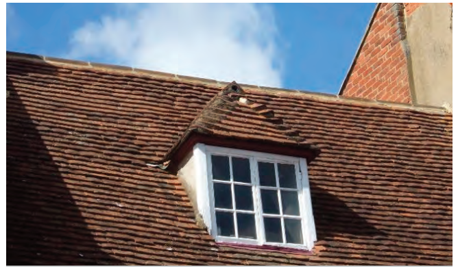
Dormer window of two 6 pane timber flush fitting casements with 'witch's eye' apotropaic detail (good luck charm) at the apex on a house in Market Square. These details are increasingly rare as window repairs / upgrades often fail to reinstate these features unless required to do so. This dormer window has slender cheeks suggesting no interventions to upgrade insulation as part of any reroofing.
