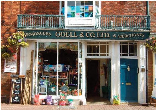
Odell's shop, High St (Grade II listed) with a 6 panel door to living quarters, a transom light with margin glazing above and ornamental cast iron railings lend distinctiveness and character to the shop front.
