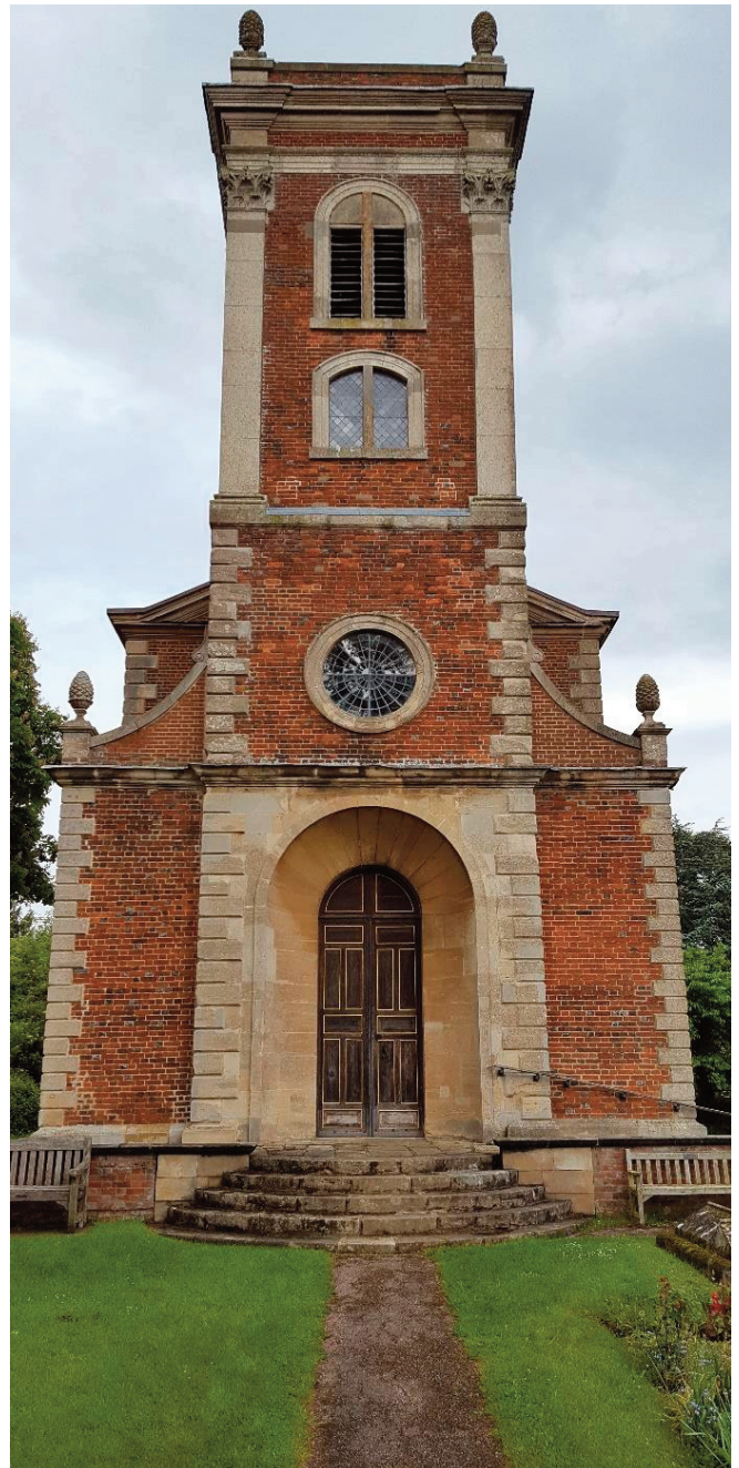
St Mary Magdalene church (Grade I listed) built principally of brick with ornate stone dressing
