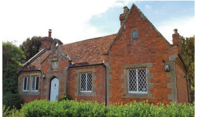
The School House - The School House (GII listed) built in brick and clay tile with ornamental stone dressing around the door and windows. The windows are metal casement in a distinctive diamond pattern.
