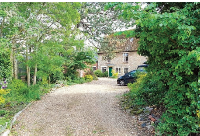
Brook Farmhouse - A view of Brook Farmhouse from the road. Note the timber side hung and flush fitting casements set under a timber lintel.
