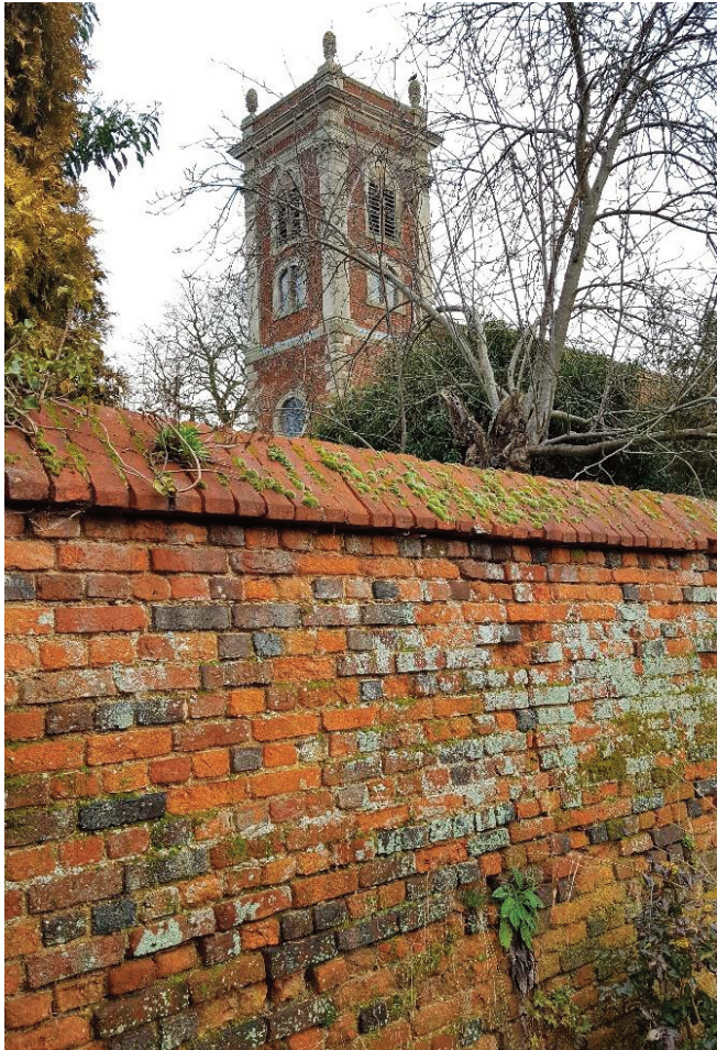
Churchyard wall - Churchyard boundary wall built in brick of varying hues using English bond – alternating courses of headers and stretchers – with triangular brick coping detail
