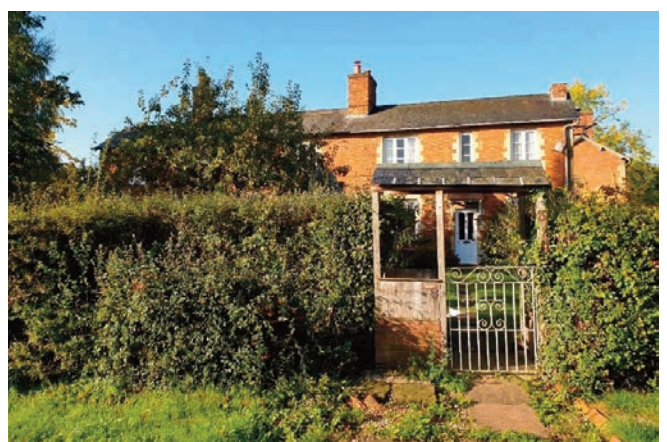
Houses overlooking Milton Road - Houses on Milton Rd of brick with stone dressing around the doors and windows. The roof is of Welsh slate suggesting a late C19th date of construction. The roof has a shallower pitch than that for clay tile.
