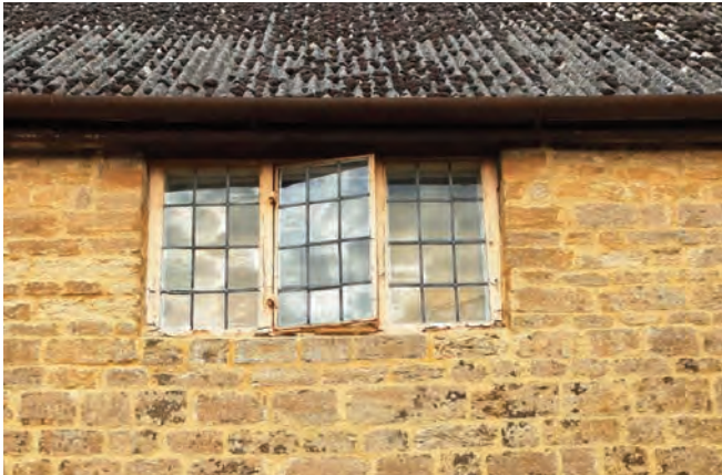
Metal casement window with a central flush fitting casement. The casement has distinctive pintle hinges. The window has no cill and sits flush with the wall exterior
