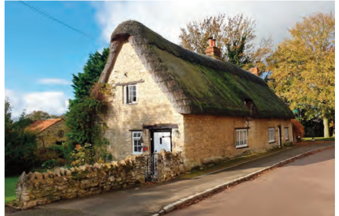
Thatch, this cottage on South Street appears to be thatched in traditional long straw thatch with its distinctive wrap around verge detail. The ridge detail is not usual for long straw and the roof would have to be sampled to confirm that it is not a hybrid form of thatching
