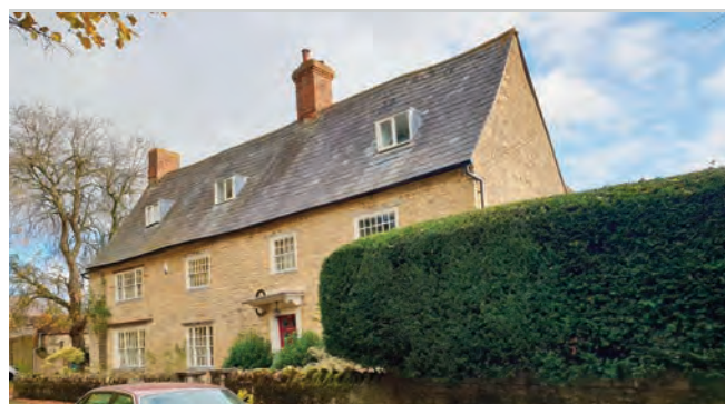
Manor Farmhouse, note the selection of window designs sitting under timber sashes rather than stone lintels. The roof is slate but the steep pitch suggests it was once thatched
