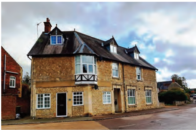
Number 5 South Street was once a shop with unusual decorative chevron stonework and carefully applied detailing to doors and windows. Unfortunately, when it was converted to solely domestic use the detailing was not as conscientiously undertaken and the building's appearance now seems slightly makeshift and unfinished
