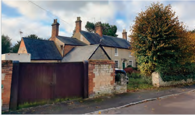
At Lime Trees farm fi red brick is used to edge walls, cope wall tops and for other incidental purposes
