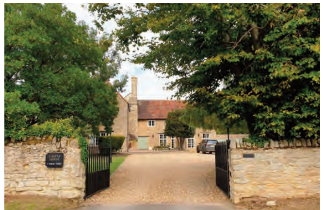
Clay tiles at Castle House, North Street. Also note the width of the front door in relation to its height
