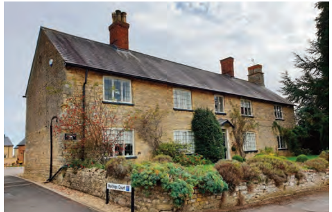
Malting farmhouse still retains a stone chimney stack, minus pots. Notice the tripartite side hung casement windows with lead comes gripping the small panes of glass into place
