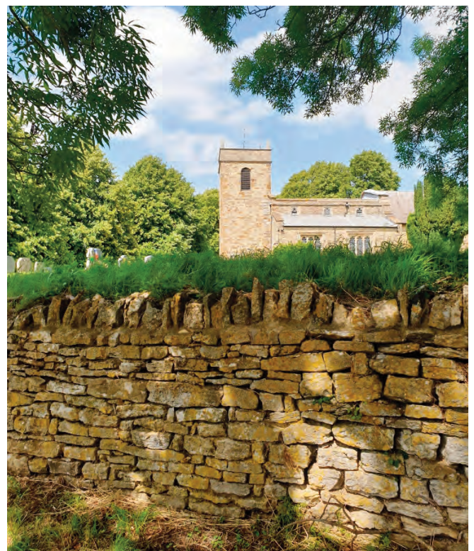
Local limestone an unpointed retaining wall on North Street with a view of the church of St Simon and St Jude beyond
