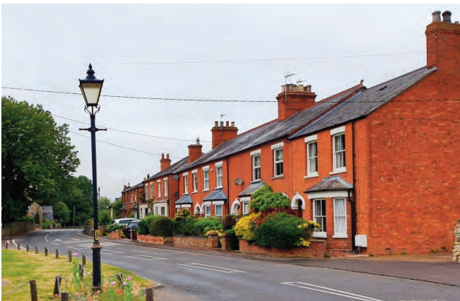
Terraced houses on North Street in red brick, dark grey slate, painted stone and timber
