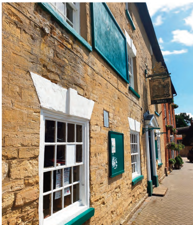
Carrington Arms with painted stone lintels over eight over eight pane timber sash windows. The windows are flush with the wall suggesting a mid, rather than late 18th century date after which windows were pushed back into their openings to discourage the spread of fire. The glass is puttied into structural timber glazing bars
