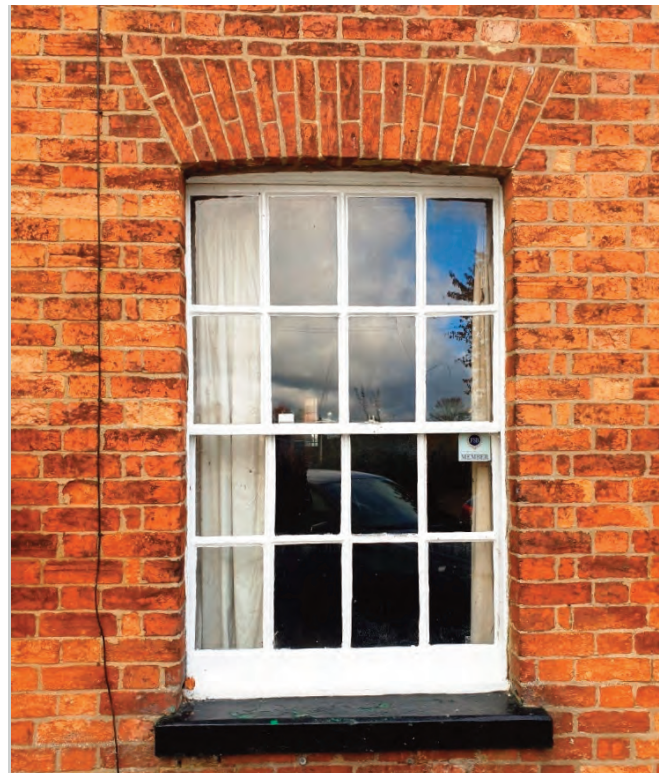
Sash window at 3 South Street under a flat head arch of gauged brickwork
