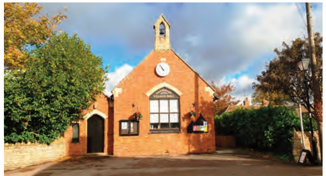
The village hall, brick with stone detailing. The brickwork is in English bond (alternating courses of headers and stretchers)
