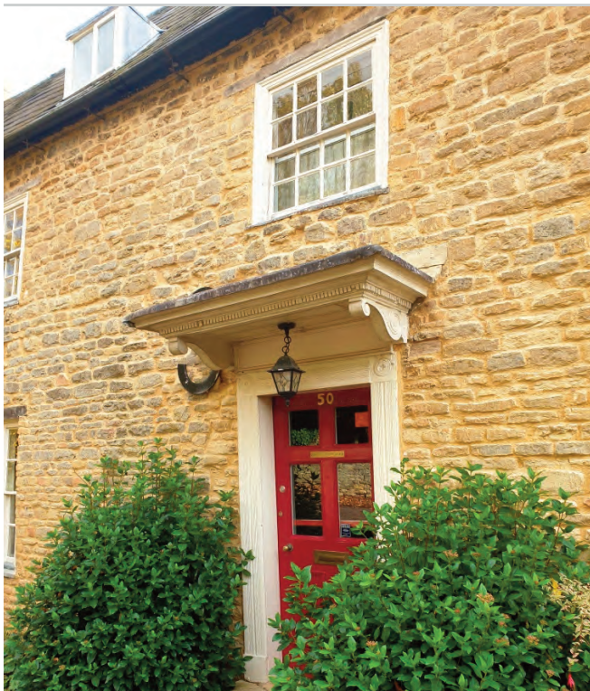
Front door details at Manor Farm adds a sense of occasion to the main entrance
