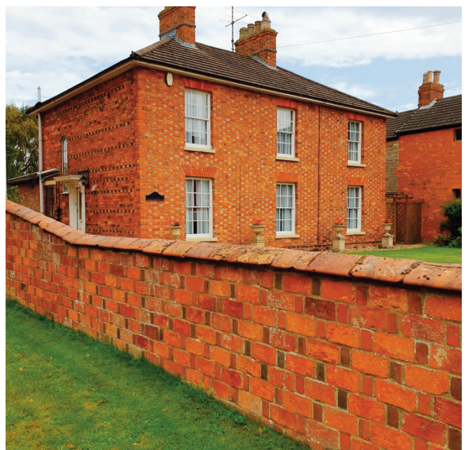
More rat trap bond in the boundary wall of Chapel House with neat terracotta coping detail. The house has a strict ornamental decorative chequer board pattern formed by alternating colours of headers and stretchers in Flemish bond. At the side are courses of stretcher brick punctuated in alternating dark and cream headers in a form of English garden wall bond. Note the six over six sash windows set into their openings and the flat head segmental arches in gauged brickwork
