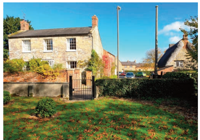
The Old Vicarage and Number 4 The Green. Two contrasting styles of stonework; the formal arrangement using carefully cut ashlar whilst the thatch cottage is of randomly coursed rubblestone
