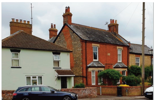
A stone building refronted in brick but the possibility that stone was a cheaper and less fashionable material for the sides of the house at the time of construction is not discounted
