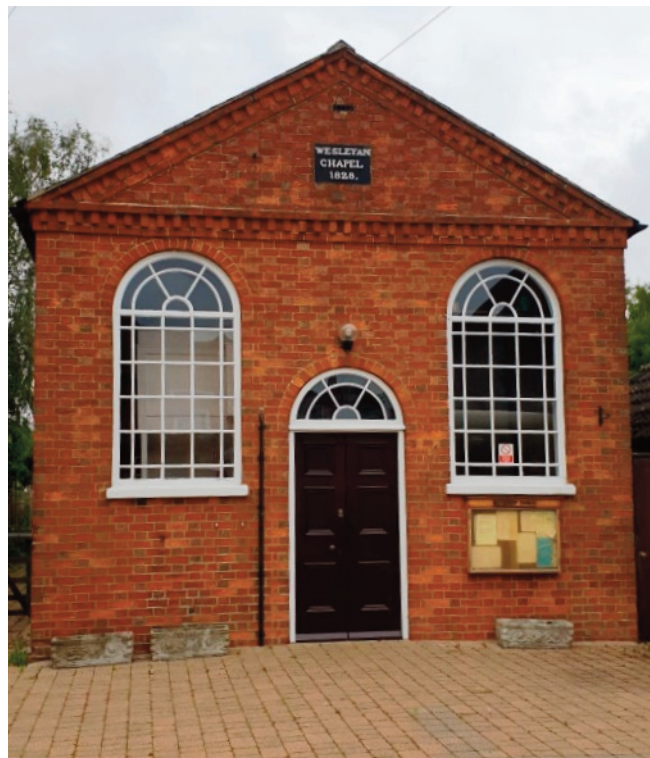
Methodist Chapel, built 1828 in flemish bond, has a pediment with dentilled eaves, delicate brick arches over semicircular arch windows that are enhanced by slim margin panes
