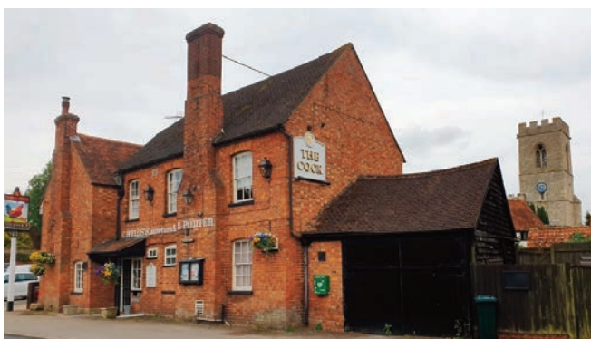
Weatherboard store standing on the west side of The Cock public house. Note the pantiled outbuilding beyond. The Cock's windows have flat head segmental arches and are set some 90mm into their opening
