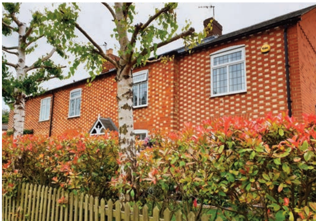
Decorative chequer board pattern made using Flemish bond, 32-34 High Street
