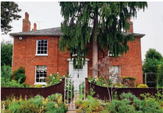
Timber doors and windows set in a symmetrical brickwork composition under a Welsh slate roof. The windows are 'six over six' timber vertically sliding sashes whilst the front door is of eight panels under a fanlight (or 'transom' light) and set within a restrained early Victorian door surround. Note the relatively small size of the door in the context of the ornamental treatment and the ornamental iron gate.
