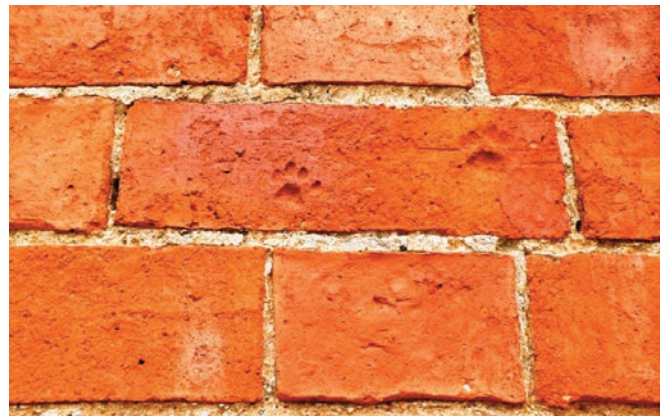
Orange brick with pawprints embedded, set in an offwhite lime and sand mortar with a little hearth grit to aid curing
