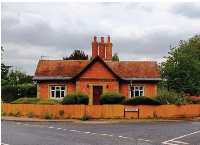
Stone dressings (left unpainted) used to enhance the presence of doors and windows, 29 High Street
