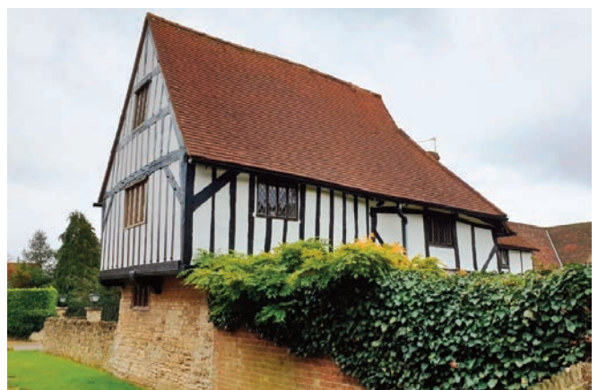
Church Farm early, cill-less, side hung, flush fitting, small pane with lead comes timber windows, set in a timber frame gable with a stone base and modern plain clay tile roof. The wall is Flemish garden wall bond
