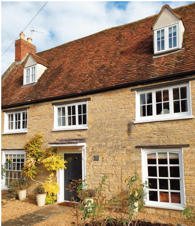
Plain clay tiles on a roof in Stoke Goldington
