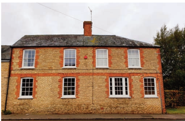
Brick detailing around the windows of 5 Berkely Close
