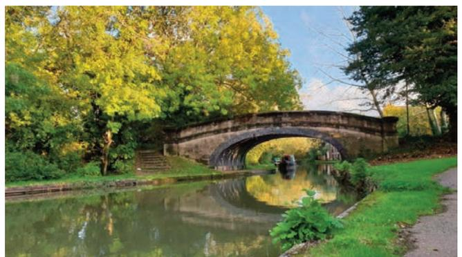
The graceful, elliptical, skewed arch of Green Bridge (Bridge 89) replaced an earlier, plainer bridge in the 1920's. The railway perfected design allows improved forward views for navigation and provides a straighter crossing line. Although the line of the canal is a man-made, superimposed feature on the landscape, dividing the Old Rectory from the village, it has become a valuable asset providing a series of accessible and attractive recreational spaces
