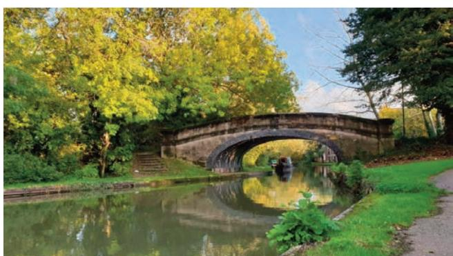
The graceful, elliptical, skewed arch of Green Bridge (Bridge 89) replaced an earlier, plainer bridge in the 1920's. The railway perfected design allows improved forward views for navigation and provides a straighter crossing line. Although the line of the canal is a man-made, superimposed feature on the landscape, dividing the Old Rectory from the village, it has become a valuable asset providing a series of accessible and attractive recreational spaces
