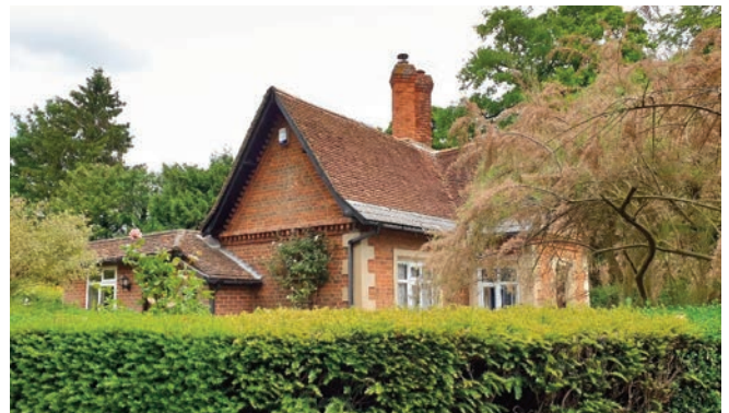
Clay tiles at Crawley Grange Lodge House, North Crawley.
