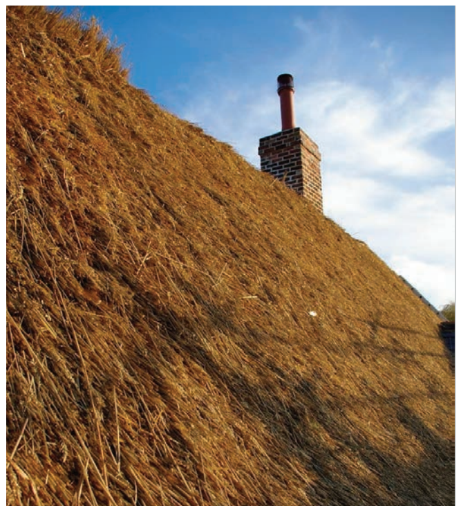
Traditional long straw thatch with ears of corn visible on the surface.
