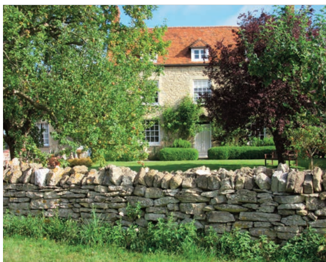
A vernacular scene at Sherington with local tile and stone. Note the open joint (mortar free) traditionally made boundary wall.
