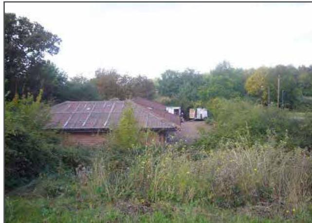
Poor quality gateway building - Horizon Training Centre
