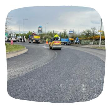
Brinklow Roundabout being resurfacing in May 2021. The surface deteriorated after a very cold, wet winter making existing defects much worse. It was resurfaced to keep the road safe for all users.
