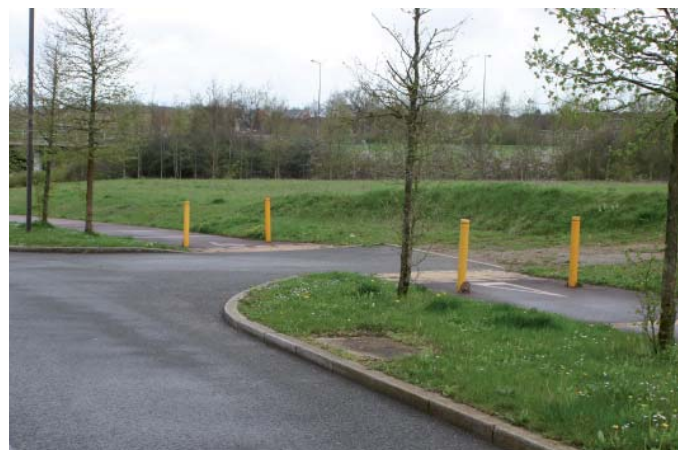
Existing bell-mouth to site off Cranborne Avenue
