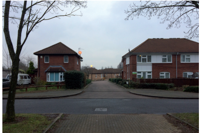
Example of level surface street access arrangement to neighbouring mews residential development
