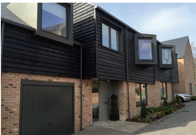
The design of the windows can add character whilst increasing surveillance and privacy
