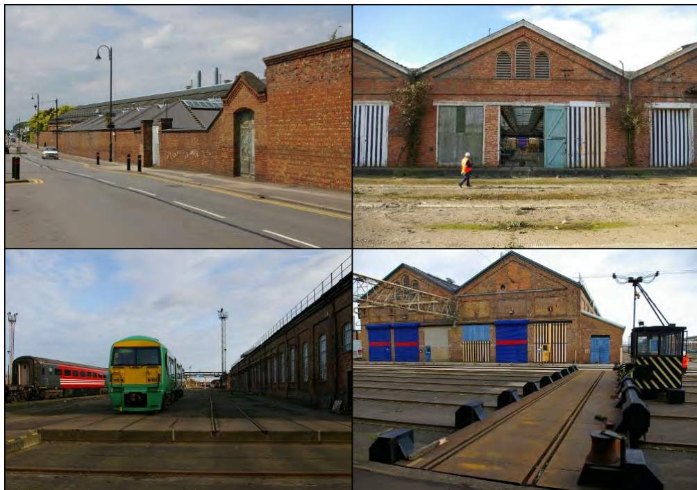
Picture 12: Views inside Railway Works site
