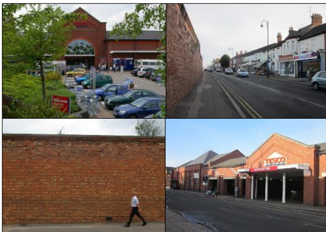
Picture 8: Views of Tesco car park below street level and pedestrian entrance-way on Stratford Road where there are steps and a ramp down to the store and car park (top left); View of Stratford Road looking east, towards Tesco showing "The Wall" (top right); "The Wall" – the Railway Work site boundary wall, Stratford Road (bottom left); View of Tesco Stratford Road entrance – a level above the store itself and The Old Bath House Community Centre (bottom right).
