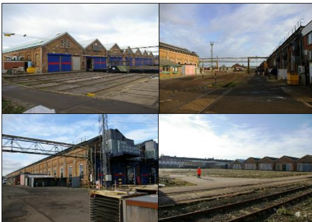
Picture 10: Views within the Railway Works site
