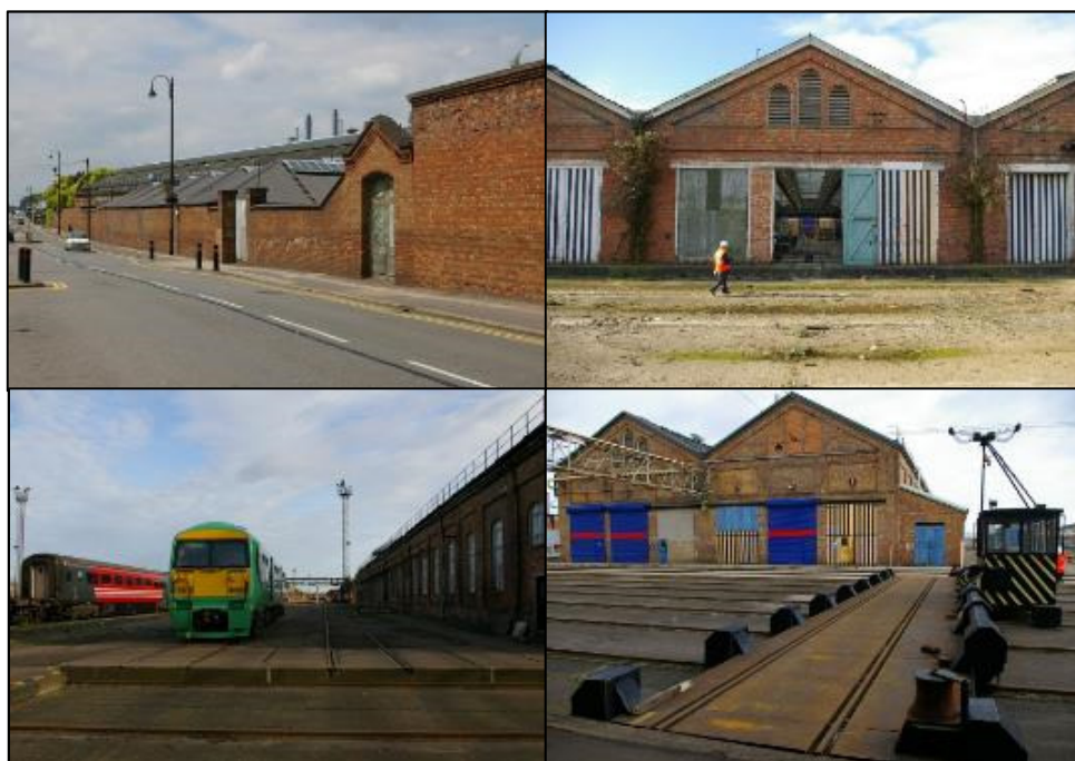
Picture 12: Views inside Railway Works site
