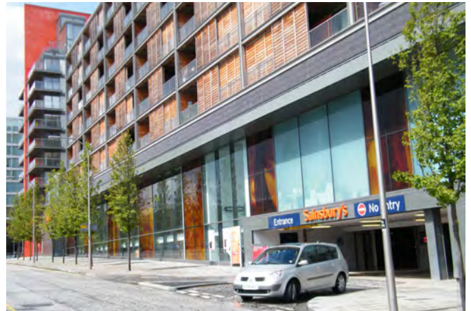
Integrated Parking Structure: Vizion development
