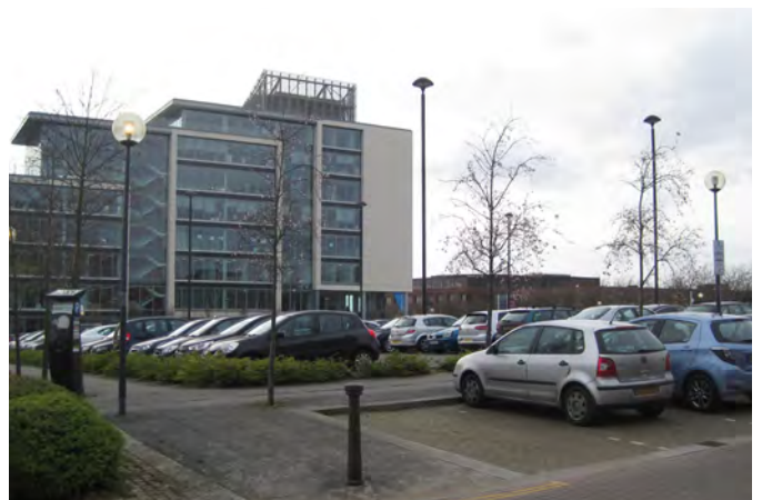
View of site from Lower Fourth Street
