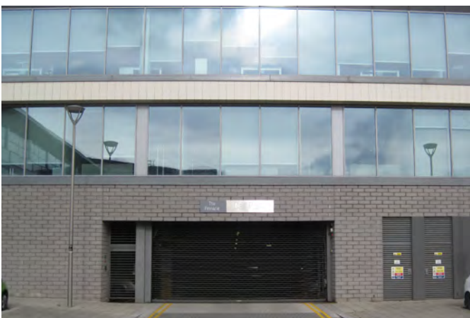
Integrated Parking Structure: The Pinnacle
