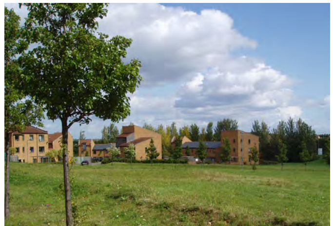
View of the site from Singleton Drive looking east.
