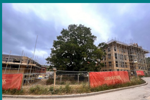
Apartment block under construction In Tattenhoe Park
