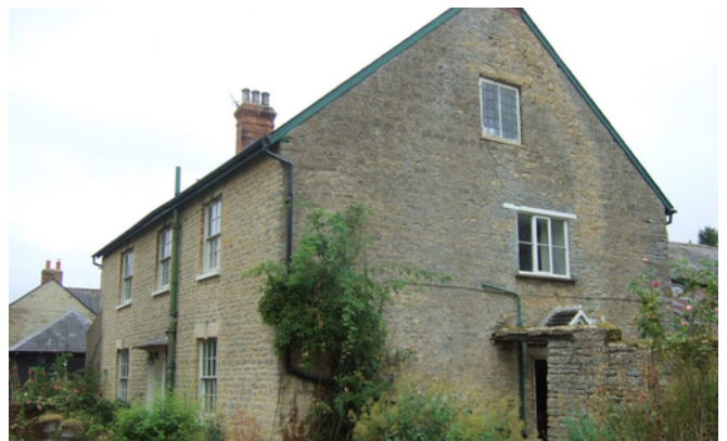
Different types of casement windows at Church Farm. Attics tended to be lit by gable windows and expensive dormer windows reserved for grander properties of the C18th.
