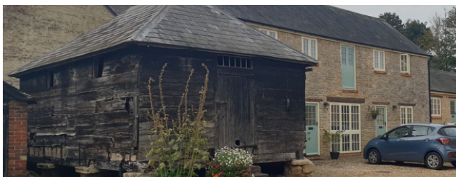
The Granary at Church Farm uses plank board as an external walling material.
