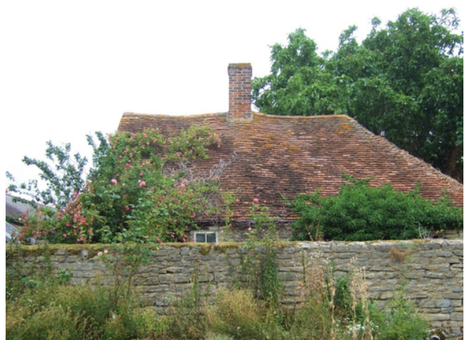
Old clay tiles
