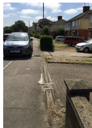
Figure 4-11: Concrete channel at the rear of public footpath
