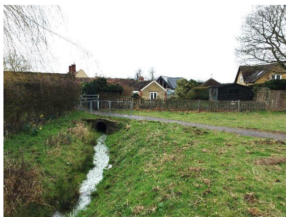
Figure 4-14: Ordinary watercourse entering culvert upstream of Stoke Goldington
