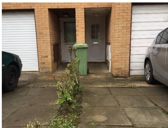
Figure 4-6: Typical low threshold of properties
