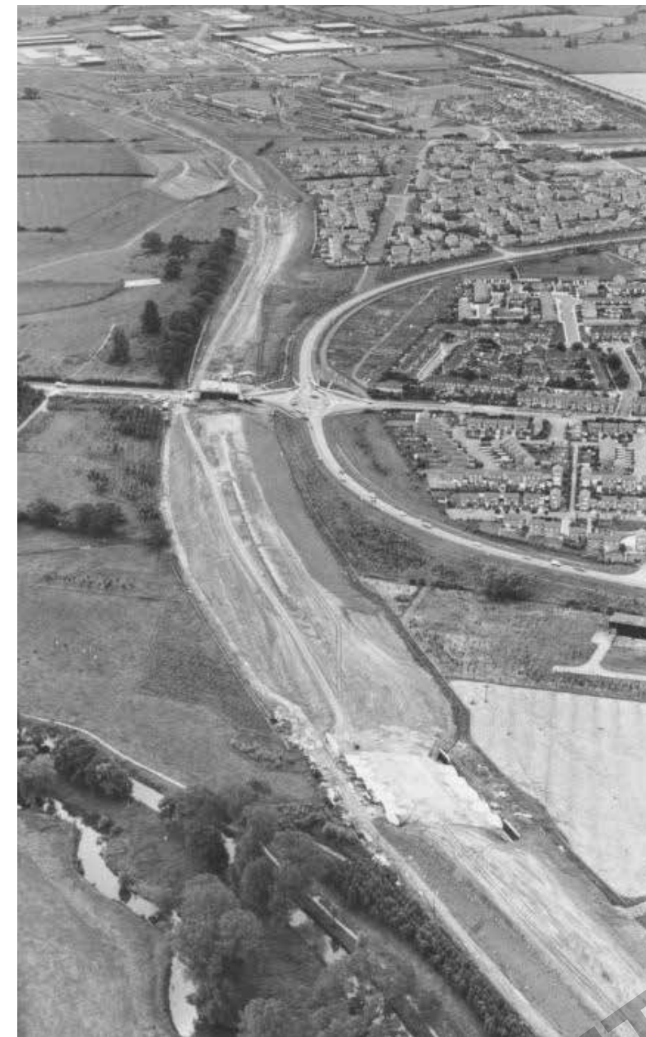
Figure 3.4 Image of the A5 under construction. Source: Milton Keynes Development Corporation
