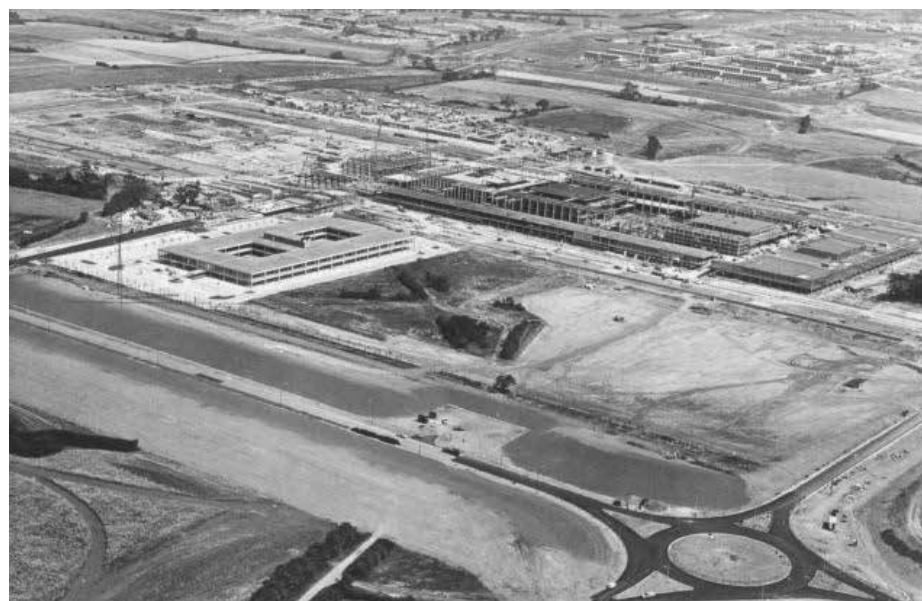
Figure 3.3 View from the north of the City Centre building site, with Lloyds Court in the foreground. Source: Milton Keynes Development Corporation
