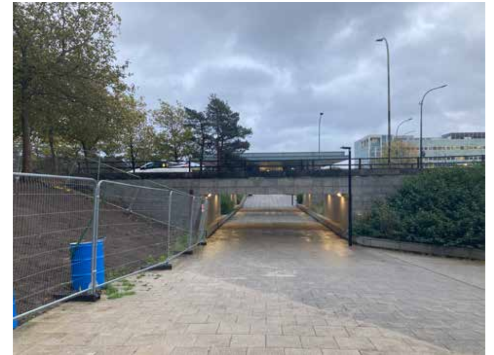
Figure 4.5 Former bus station (looking south)
