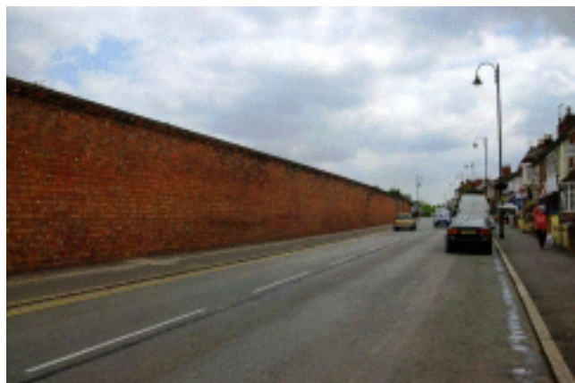
Picture 2.2 The works boundary wall
