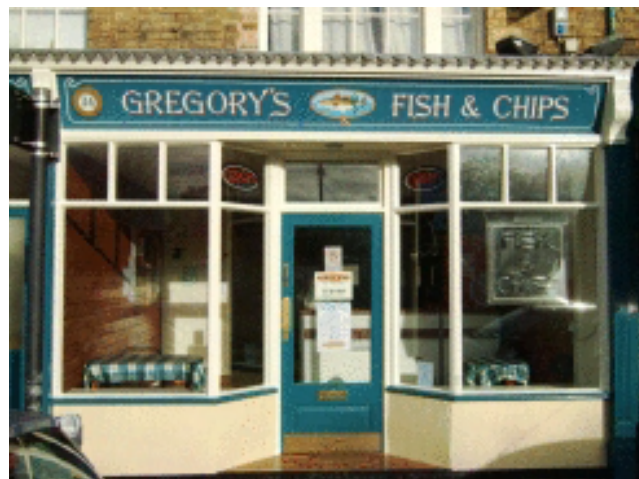
Picture 2.49 Refurbished shop front, Church Street
