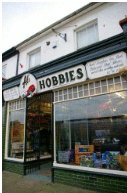
Picture 2.113 A well maintained, retained shop front on Stratford Road
