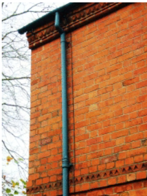
Picture 2.69 Iron down pipe, Buckingham Street
