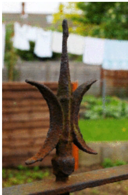
Picture 2.70 Finial detail on railing fronting Green Lane
