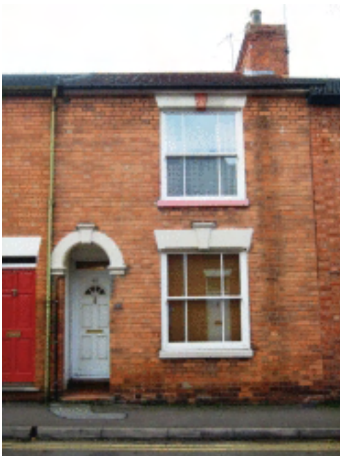
Picture 2.63 A simple terrace (Radcliffe Street) with large windows allowing just enough room for the ceiling joists between ground and first floor.
