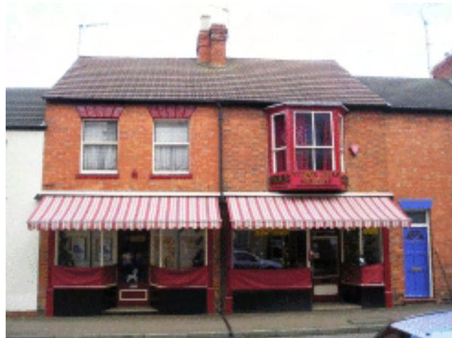
Picture 2.74 Shop with awnings and timber canted bay window to upper floor
