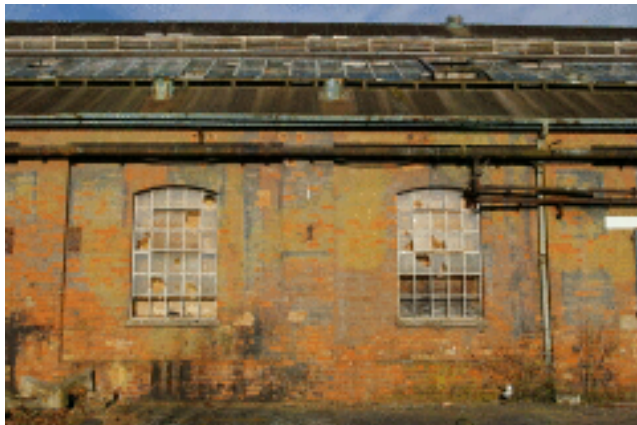
Picture 2.21 Faded camouflage on works buildings
