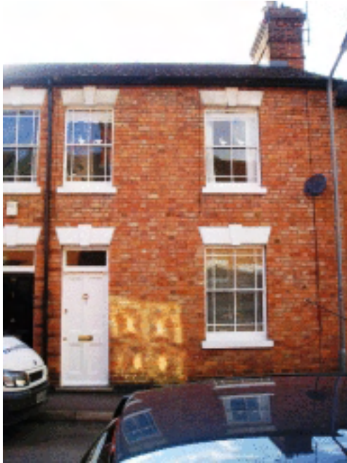
Picture 2.60 A plain terrace on Radcliffe Street. This design relies on windows for its architectural voice. Elsewhere, however, windows have been replaced with much less eloquent alternatives however.
