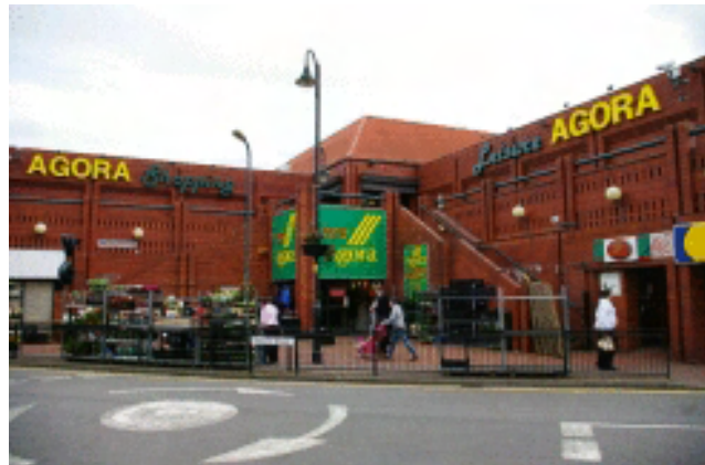
Picture 2.108 The Agora Centre, Church Street
