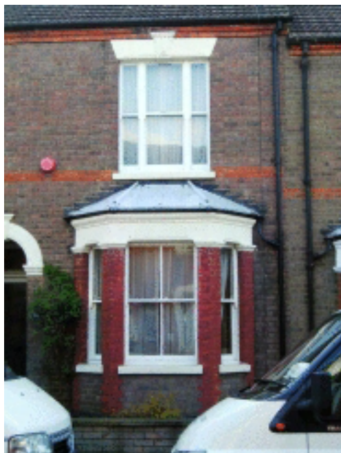
Picture 2.82 Tripartite window above lead roofed canted bay window, Cambridge Street
