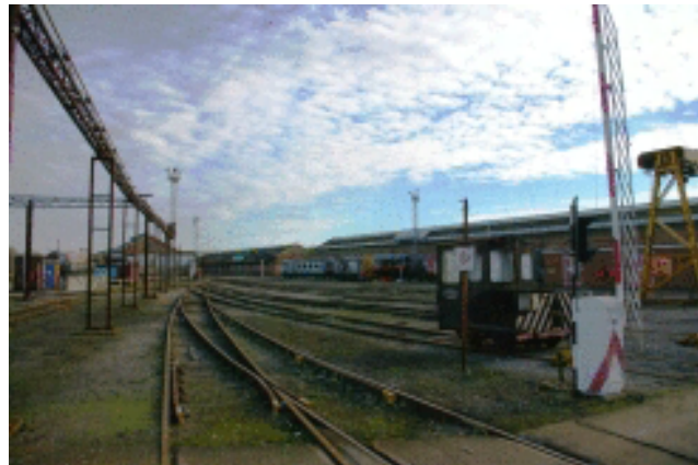
Picture 2.23 The western end of the works site
