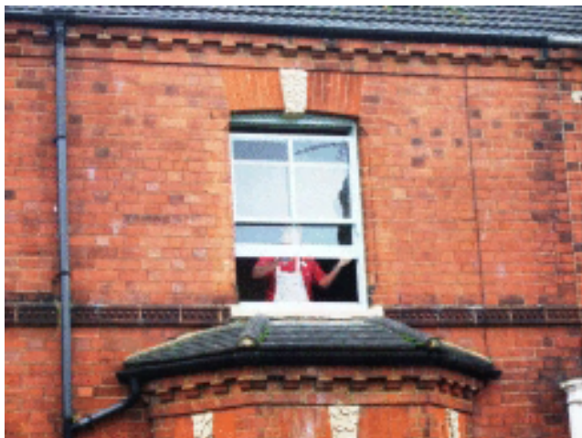
Picture 1.8 Timber sash being repaired
