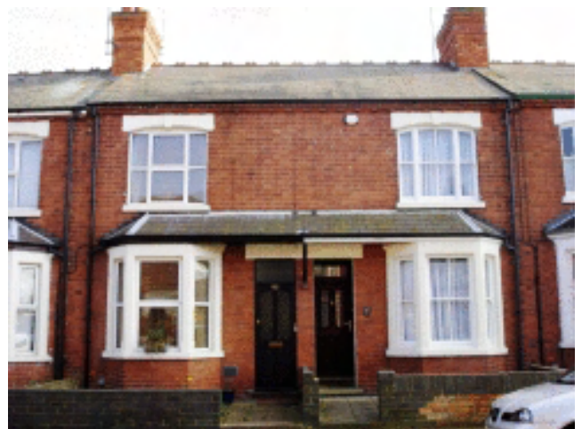
Picture 2.81 Houses on Western Road.
