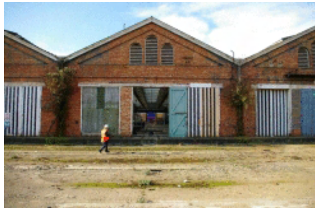
Picture 2.37 Three light detail in gable ends and ledged and braced doors
