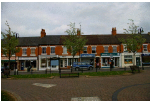
Picture 2.12 East side of The Square
