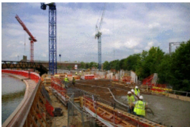
Picture 2.112 Work underway on the Wolverton Park site
