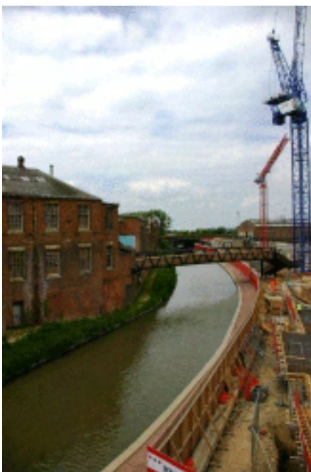
Picture 2.31 Redevelopment taking place opposite The Triangular Building. Stephenson's Bridge can be seen in the background behind the new footbridge
