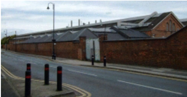
Picture 2.18 Wolverton works stop abruptly along the line of the Stratford Road boundary wall
