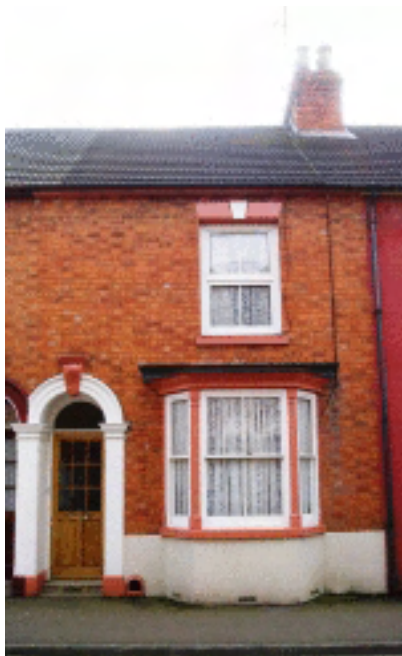
Picture 2.65 Surviving timber canted bay window, Aylesbury Street
