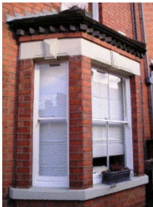
Picture 2.84 Victorian sashes in a simple but elegantly detailed canted bay
