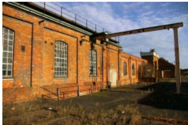
Picture 2.36 Iron windows set in pier and panel construction
