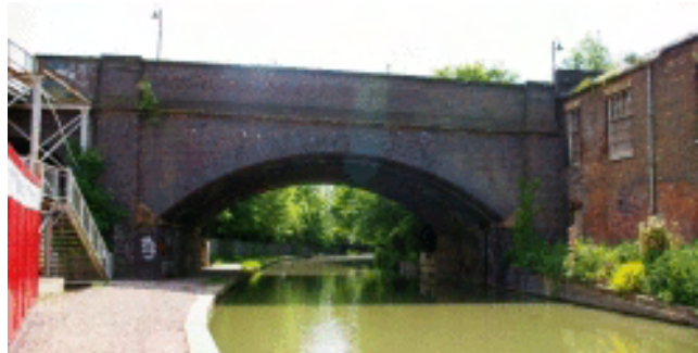
Picture 2.32 The Stratford Road bridge
