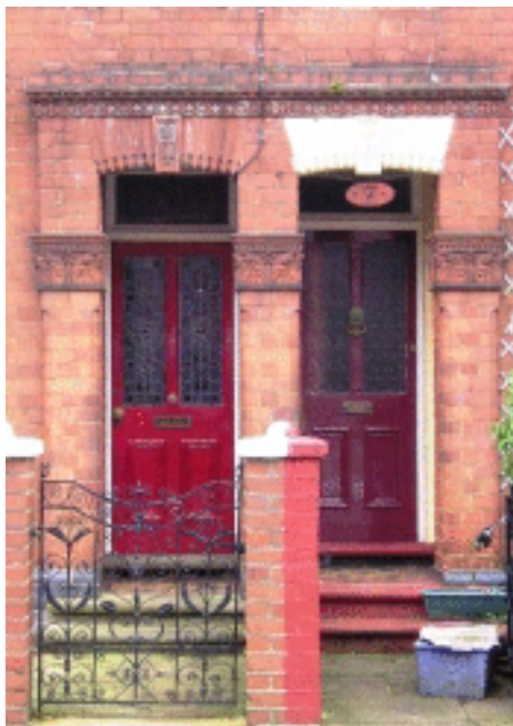
Picture 2.85 Doors, Victoria Street. Note the ornamental gate on the left side
