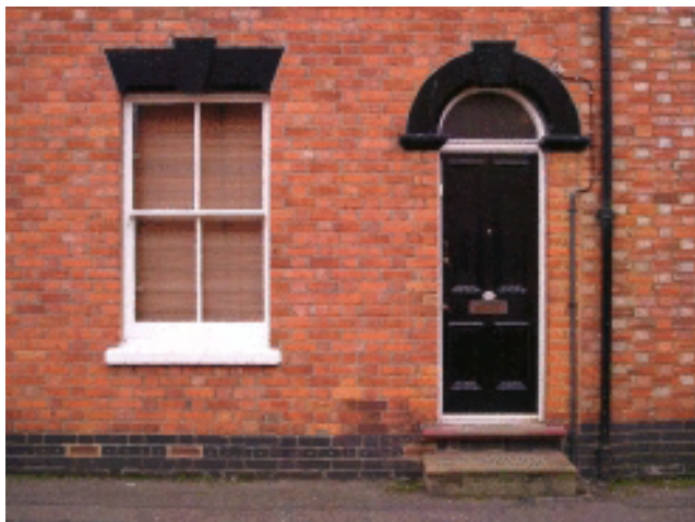
Picture 2.66 Door and window detail showing both recessed from the front of the property by about the width of a brick (note also the blue brick plinth and cast iron drain pipe)
