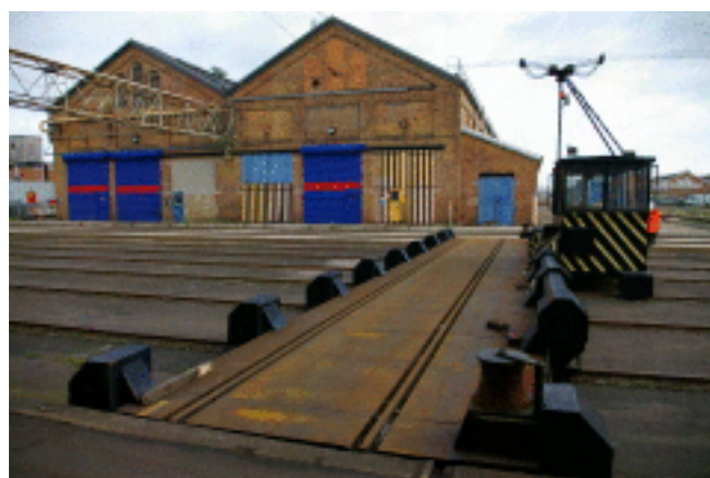
Picture 2.24 A works traverser
