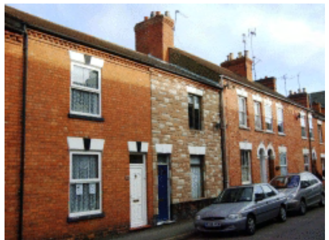
Picture 3.8 Stone cladding is harmful to the appearance and fabric of individual terraces. It causes the eye to be drawn to a discordant alteration at the expense of authentic character
