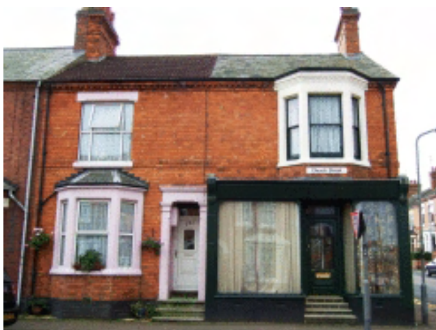
Picture 2.73 Shop front with canted bay windows above
