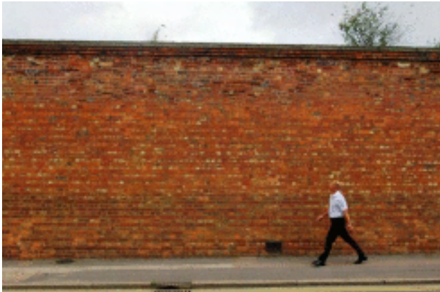
Picture 2.38 Works boundary wall
