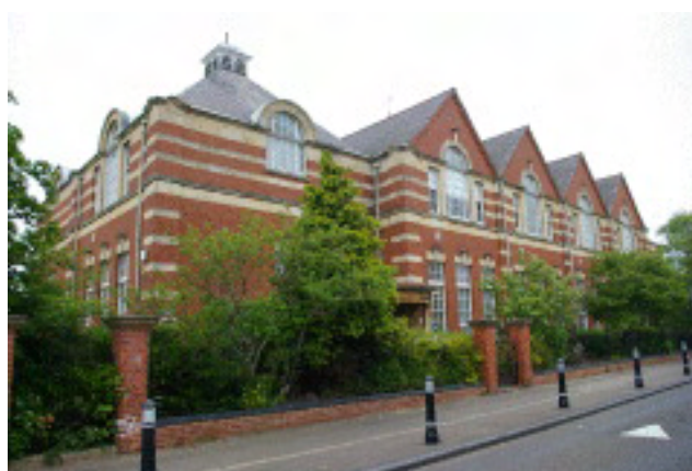
Picture 2.15 Wyvern School - South Block
