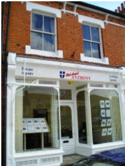
Picture 2.47 A well maintained shop front on The Square
