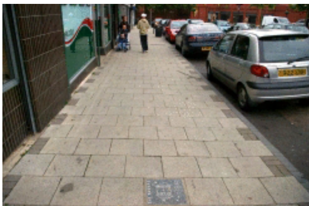
Picture 3.11 New surfacing in The Square
