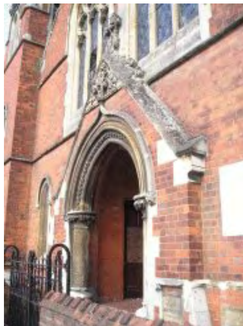
Picture 1.6 Brick with stone ornamentation at the Wesleyan Chapel
