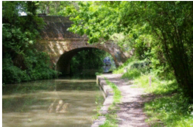
Picture 1.4 Bridge 69, Grand Union Canal
