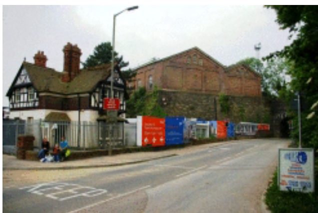
Picture 2.34 The eastern approach to Skew Bridge with the Keepers Lodge in the foreground and the Royal Train Shed above
