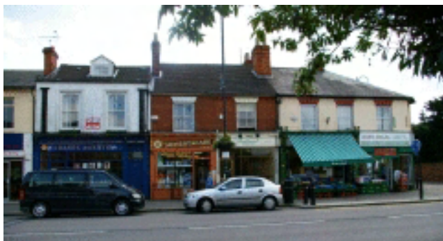
Picture 2.3 Commercial premises on the south side of Stratford Road
