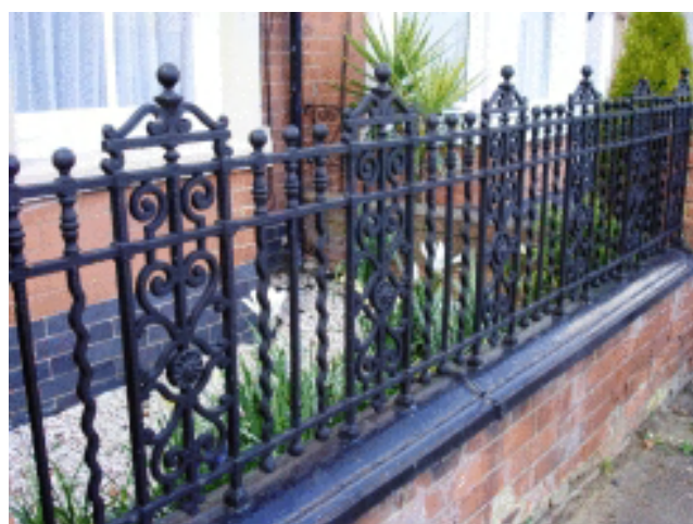
Picture 2.87 Original railings on a boundary wall in Cambridge Street
