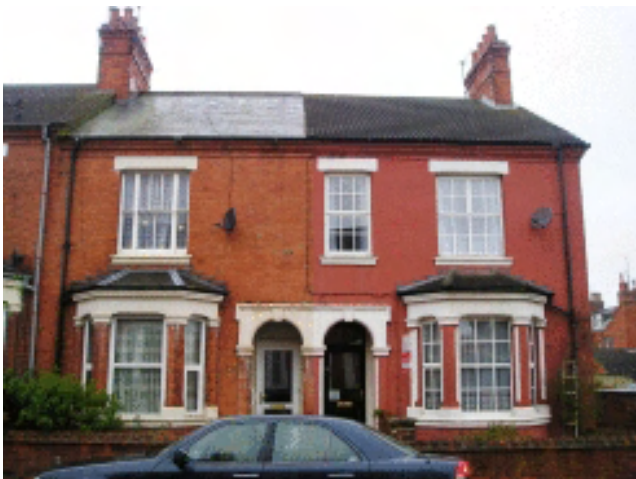
Picture 3.9 Substantial investment for maintaining property is evident. However, poor advice and selection has led to numerous mismatched alterations. Across the conservation area this process has fractured the shared architectural language of the terraces
