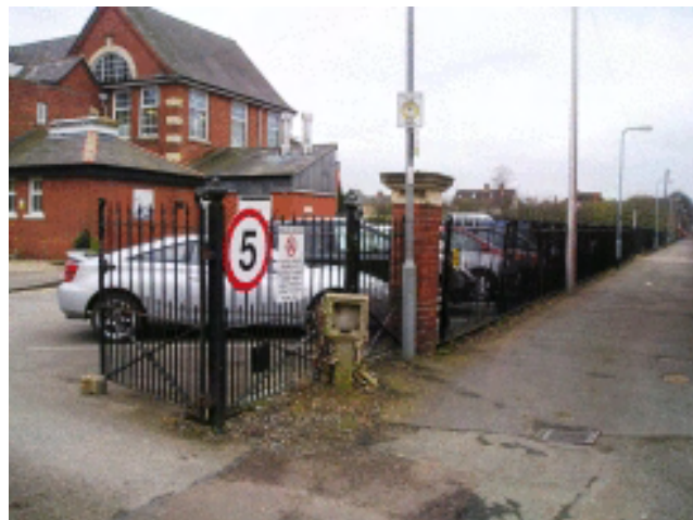
Picture 2.101 A lengthy run of iron railings commences at the entrance to Bushfields Middle School
