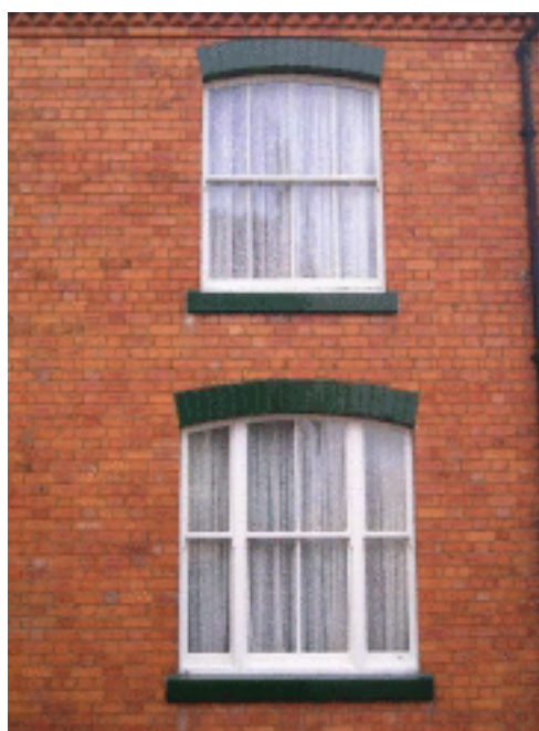
Picture 2.110 Neatly detailed domestic window arrangement
