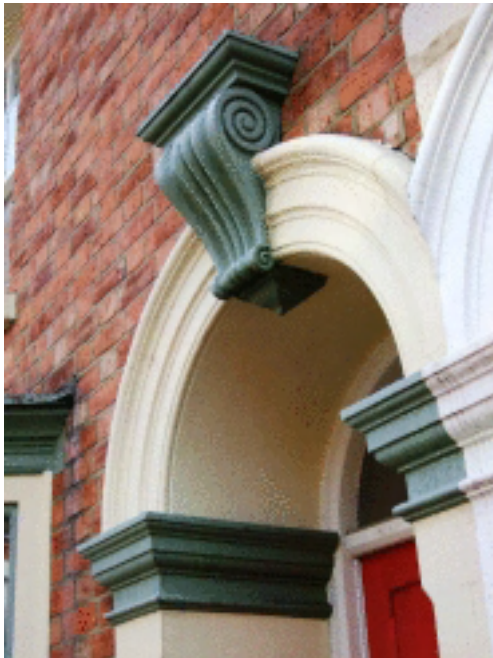
Picture 3.6 Decorative console detail, Buckingham Street. Originally this detail would probably have been left unpainted.
