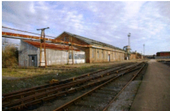
Picture 2.20 Former works buildings
