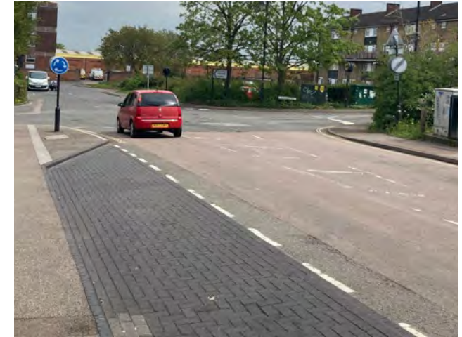
Figure 35: Differentiated surfacing treatment of the parking bays.
