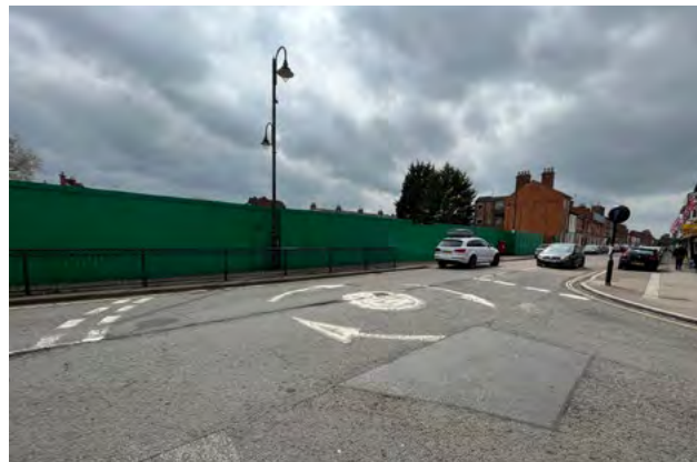
Figure 32: Low quality, well-worn road surfacing and markings at the roundabout of Church Street and Radcliffe Street.
