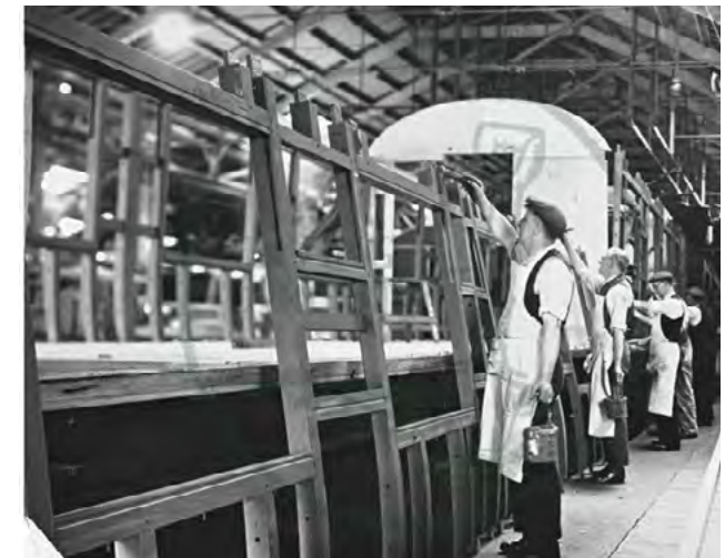
Figure 05: The Wolverton Railway Works Paint Shop.
