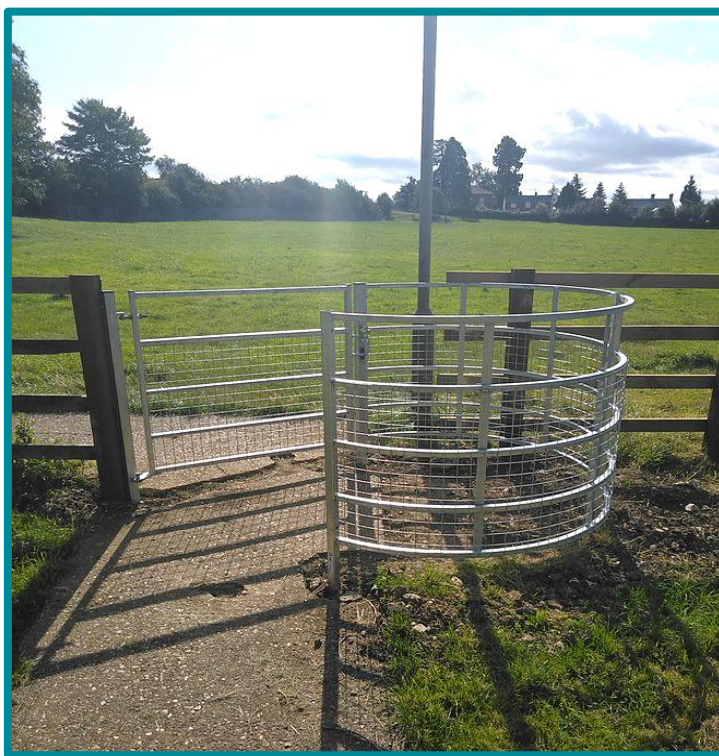
Figure 14. Large accessible kissing gates can be used by those with some mobility scooters, and pushchairs
