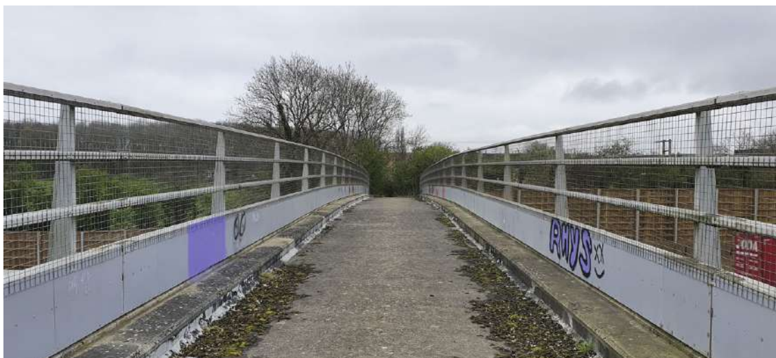
Figure 2-3: Existing bridge over the M1
