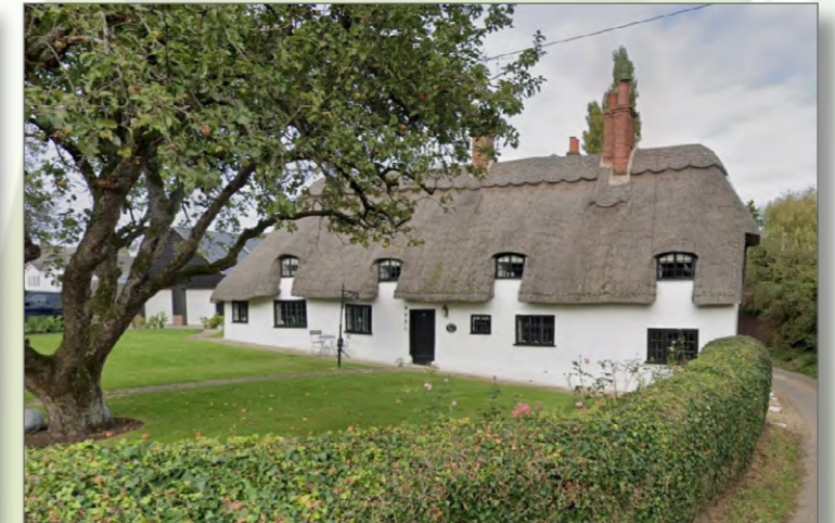
Fig no. 21, Photo of Grade II Listed Cross End Cottage.
