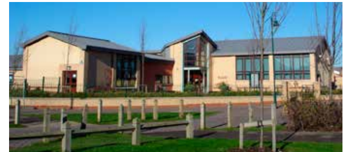
Above: Community building, Hampton, Peterborough
