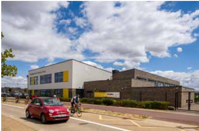
Above: Cyclists passing Brooklands Farm Primary School, Milton Keynes
