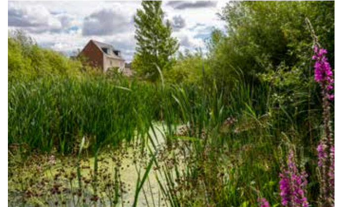
Above: Sustainable drainage features, Brooklands Meadows
