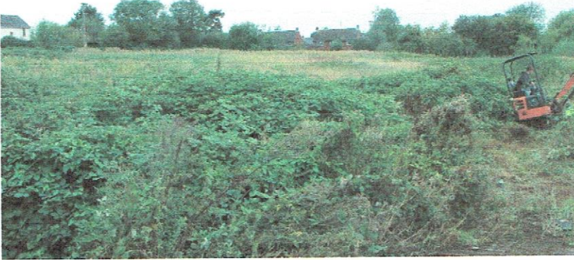
Photo No.2 Example of excavating a stable platform.
