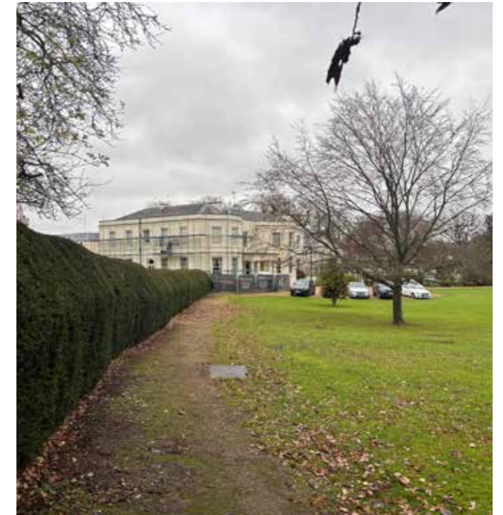
Figure 4.7 Southern elevation of Wavendon House December 2025
