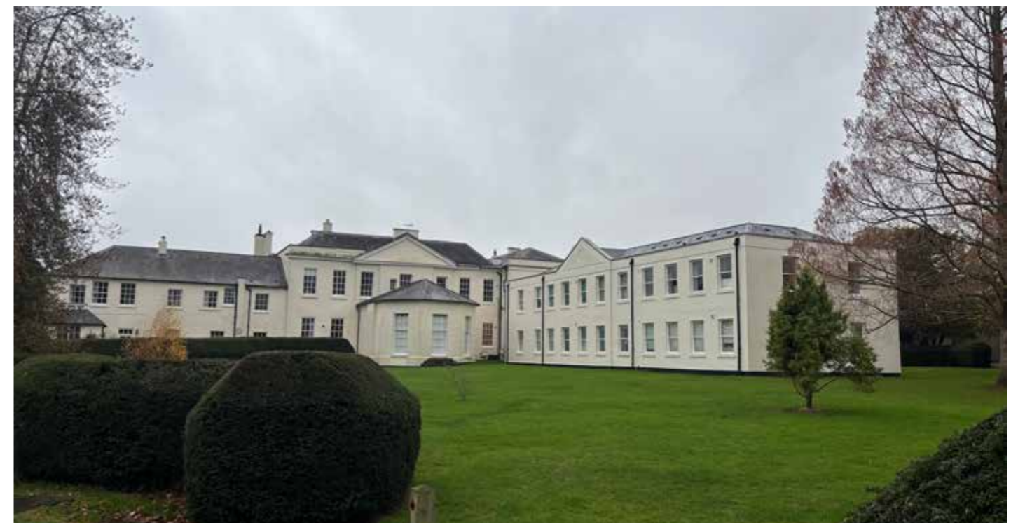
Figure 4.8 Original primary elevation (north facing) which later became the rear elevation following the expansion under Hoare. Note the central canted bay extension under the pediment December 2025
