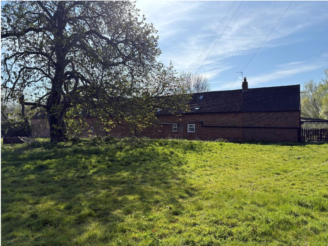
Plate 36 Looking south to the rear elevation of 3, 5, 7, and 9 Cross End
