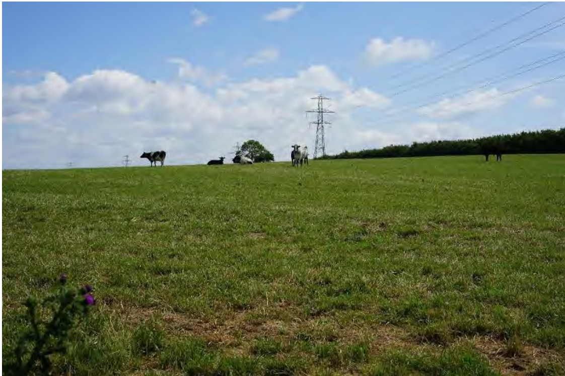
Image EDP 3.8: Prominent high voltage pylons and overhead powerlines located within the Site.
