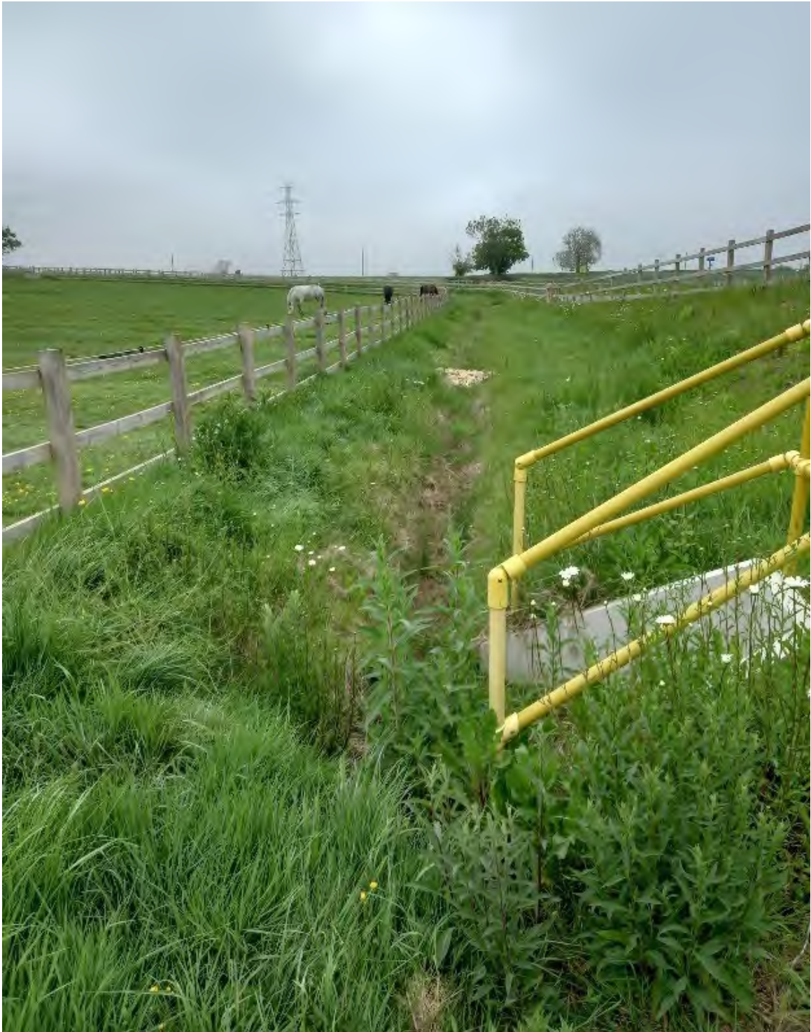
Image EDP 3.13: A swale adjacent to the central access road.
