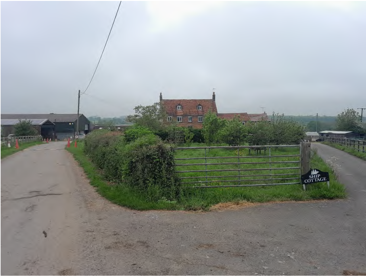
Image EDP A1.3: North-west facing view towards Grade II listed Lower Salden Farmhouse ( 1288667 ) from the trackway to the farm. Image shows the farm's front garden and orchard setting elements with its rear farmyard complex to the rear and extending round to the west and east sides.
