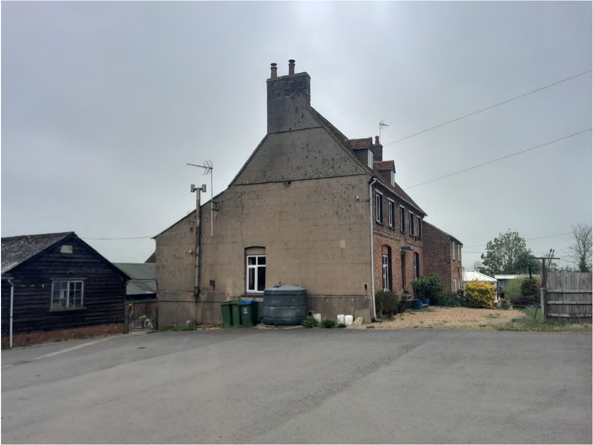
Image EDP A1.2: North facing view of the west side elevation to the Grade II listed Lower Salden Farmhouse (1288667). West side elevation features a rendered west gable wall. Image also shows rear 19 th century lean-to extension as well as its immediate front garden and west side and rear farmyard complex setting.
