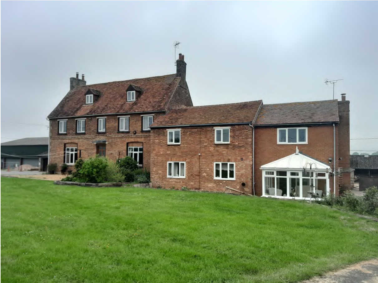
Image EDP A1.1: West facing view of Grade II listed Lower Salden Farmhouse ( 1288667 ) and its modern adjoining 20 th century extensions on its right side within its front garden setting.
