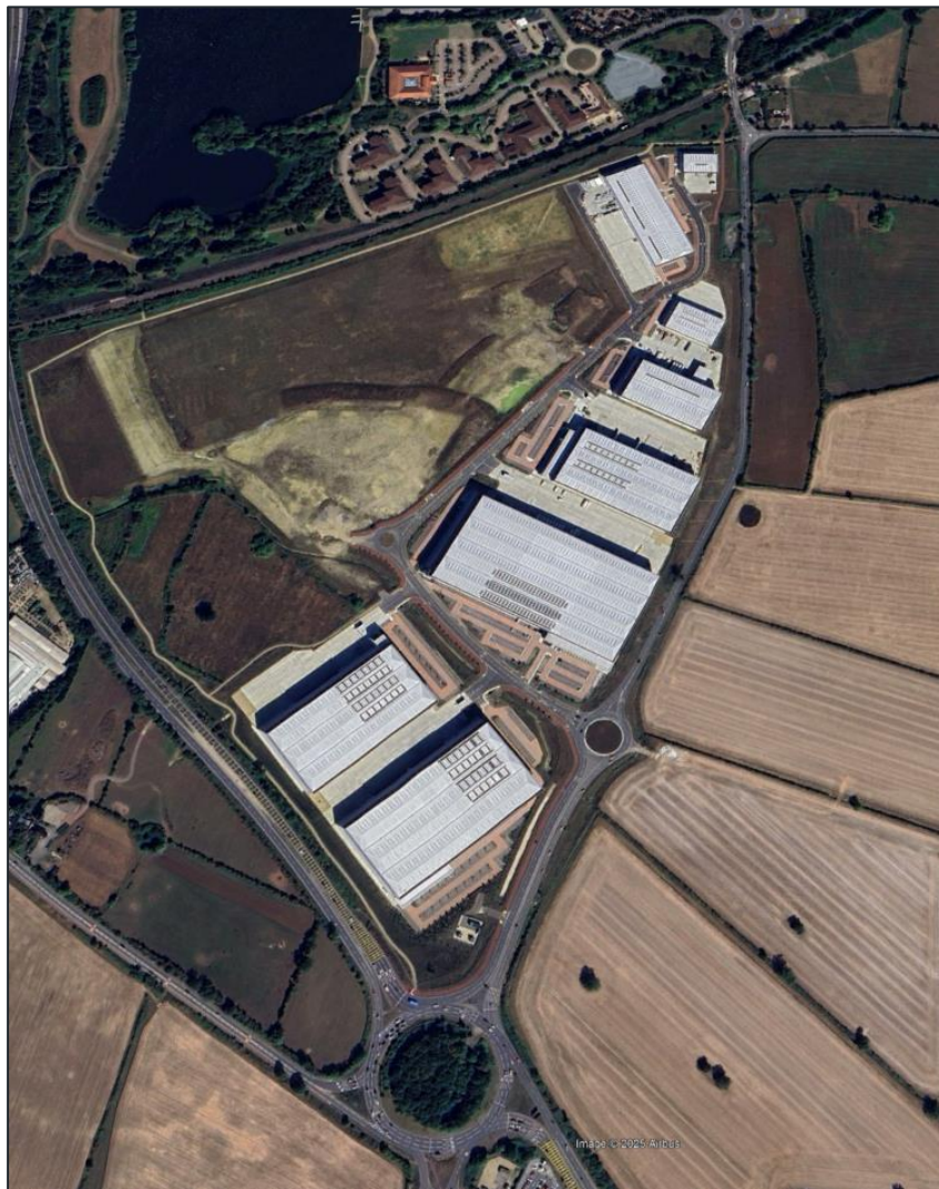
Figure 2-11 – Redway Through South Caldecotte Development
