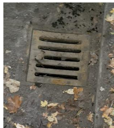
Example footway gully
