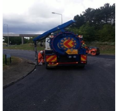
Gully Tanker cleaning a gully on a roundabout
