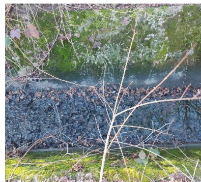
E.g., Ditch cleaned by Ditching bucket
