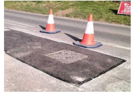
E.g., Manhole cover in typical situation in road
