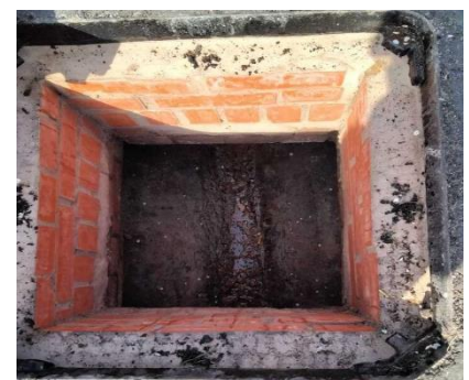
E.g., Access point showing the pipe within chamber
