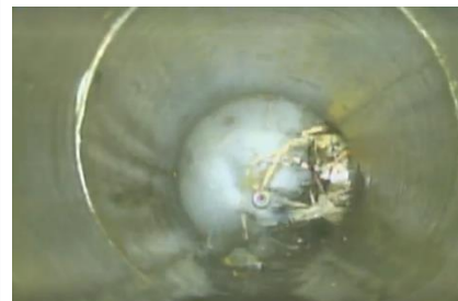
E.g., Root cutting In Progress to remove roots from pipe
