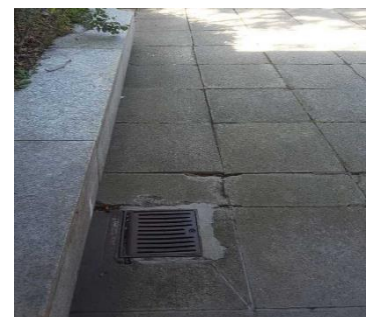
E.g., Footway Gully in underpass
