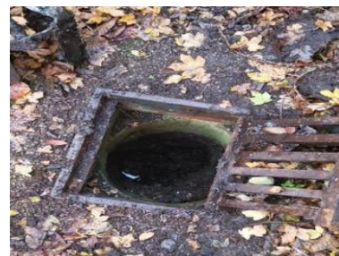
E.g., footway gully in the process of handcleaning
