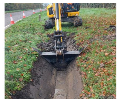
New ditch or heavily silted ditch being recut by V bucket
