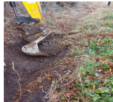
E.g., Ditch cleaned by Ditching bucket
