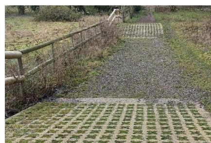
E.g., Concrete Bunds/ Soil Bunds Old farm Park Track – Stoke Goldington
