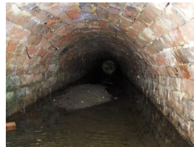
E.g., Brick Arch Culvert Cranfield Road -North Crawley
