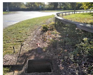
e.g., access chamber to catchpit on grid road
