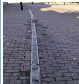
E.g., ACO channel in block paving.
