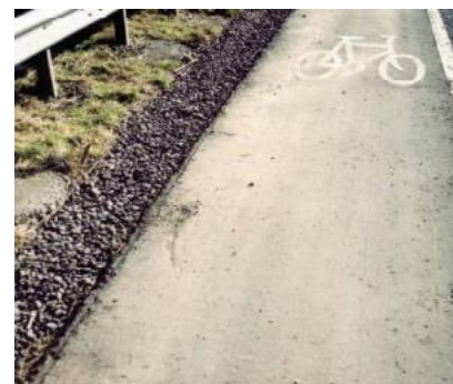
E.g., Filter drainage by roadside
