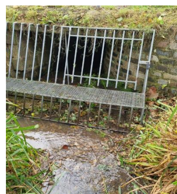
E.g., Trash Grill cleaned
