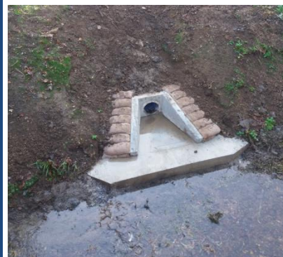
E.g., Concrete Head wall -
