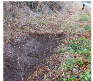
E.g., Ditch being cut
